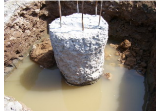
FIG. 1. Grouted gravel pile head after excavation.
