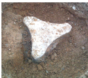
FIG. 1. Cross section of Y-pile.
