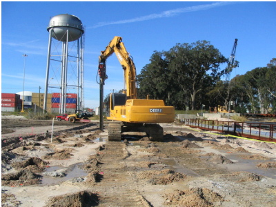
(b) Vibratory compaction at CB8 of Savannah Port
