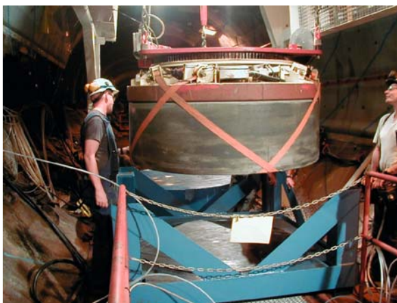
Fig. 5.16 Placement of a 2000 kg buffer block of MX-80 bentonite in a deposition hole [1]
