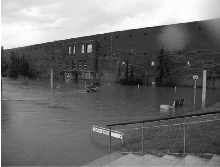
FIGURE 6.12 Flooding, Greve 2002—before adaptation to climate changes. (From DANVA, Urban Climate Change [Original title: En koge bog for analyser af klimaændrings effekter på oversvømmelser i byer], 2011.)
