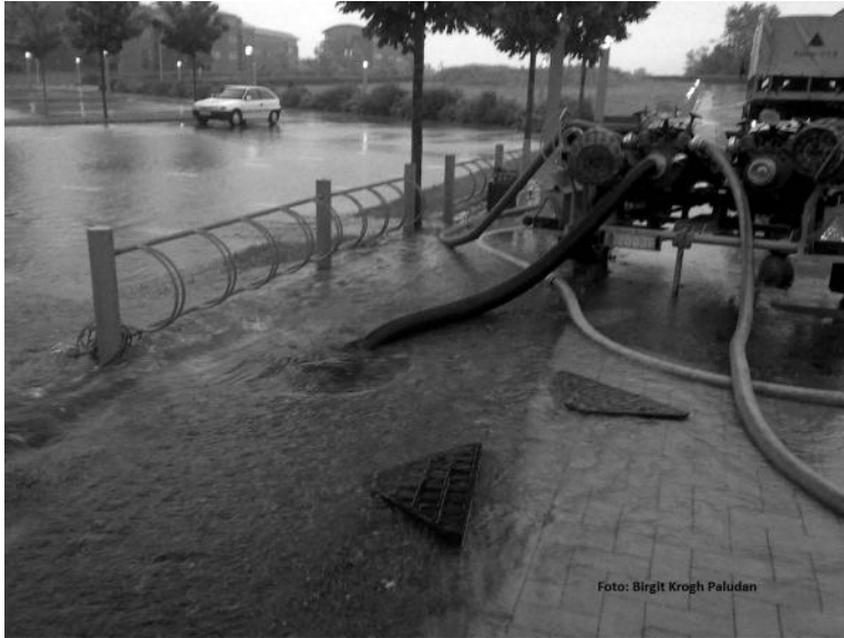
FIGURE 6.11 Mobile pump used at Greve Gymnasium during extreme rainfall in Greve on July 5, 2010. (From DANVA, Urban Climate Change [Original title: En kagebog for analyser af klimaændringers effekter på oversvømmelser i byer], 2011.)
