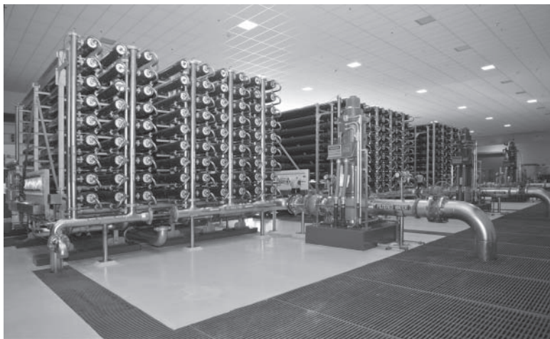
Figure 9-2 Typical reverse osmosis facility.
