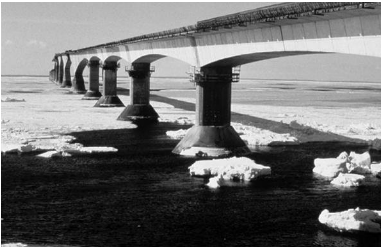
FIGURE 2.3 Confederation bridge (Canada) still under construction. (From Bercha Group, Homepage of Bercha Group, Consulting Services Since 1975, http://www.berchagroup.com/ , 2012. With permission from Frank Bercha, Bercha Group, Calgary, Canada.)
