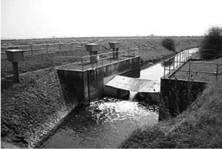
FIGURE 4.11 Crump weir on a stream.
