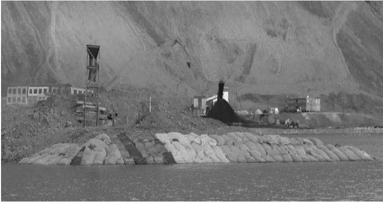
FIGURE 2.2 Testing the use of geobags to reduce erosion at Svea Mine, Spitsbergen. (Reproduced from Caline, F., Coastal sea ice action on a breakwater in a microtidal inlet in Svalbard, PhD thesis, NTNU, Trondheim, No. 226, October 2010.)
