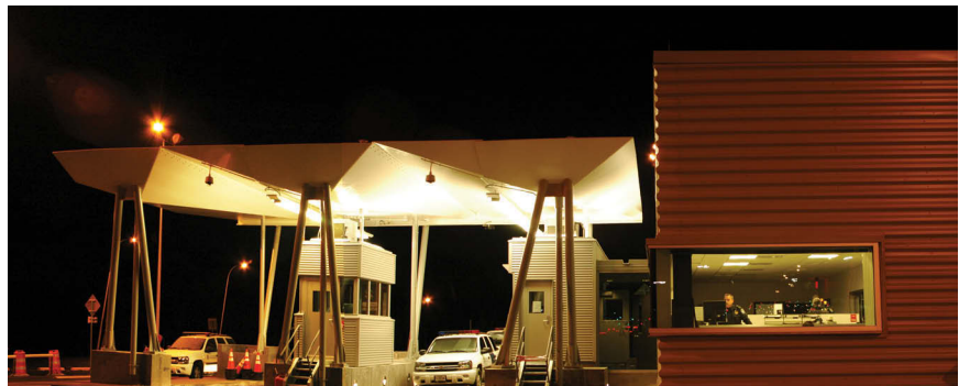
opposite: Folded steel canopy at passenger inspection
