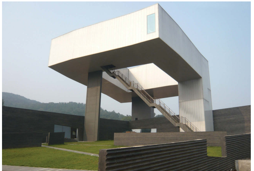
bottom: View of courtyard with "floating gallery" above
