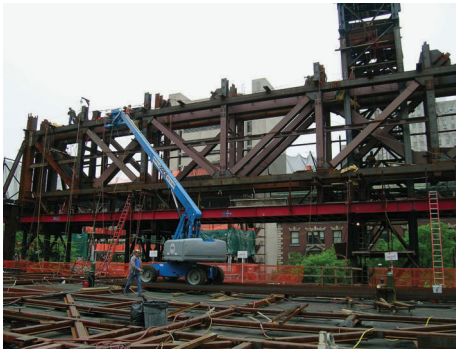
fig. 4 | Construction view; trusses span width of gymnasium
