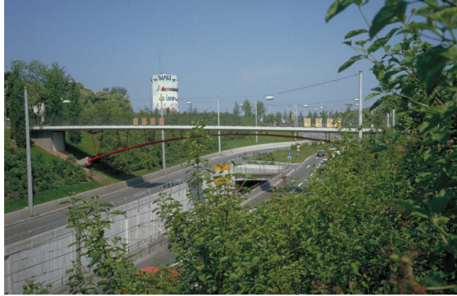
figs. 6, 7 | The inversion of a suspension bridge results in an arch bridge, Pragsattel I, by SBP, Stuttgart, Germany, 1992
