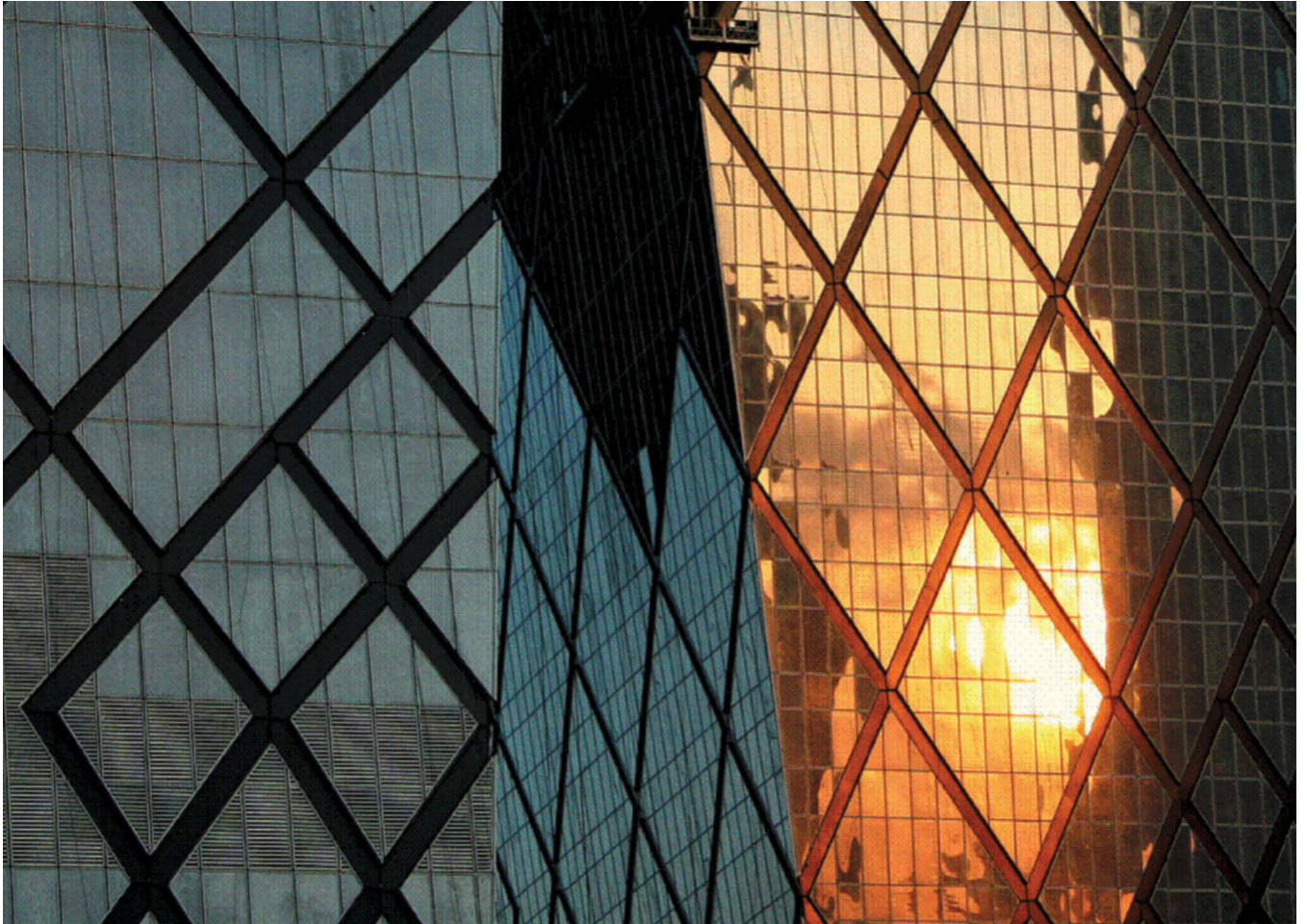
fig. 1 | China Central Television (CCTV) Headquarters, by Office for Metropolitan Architecture (OMA), Beijing, China, 2010
