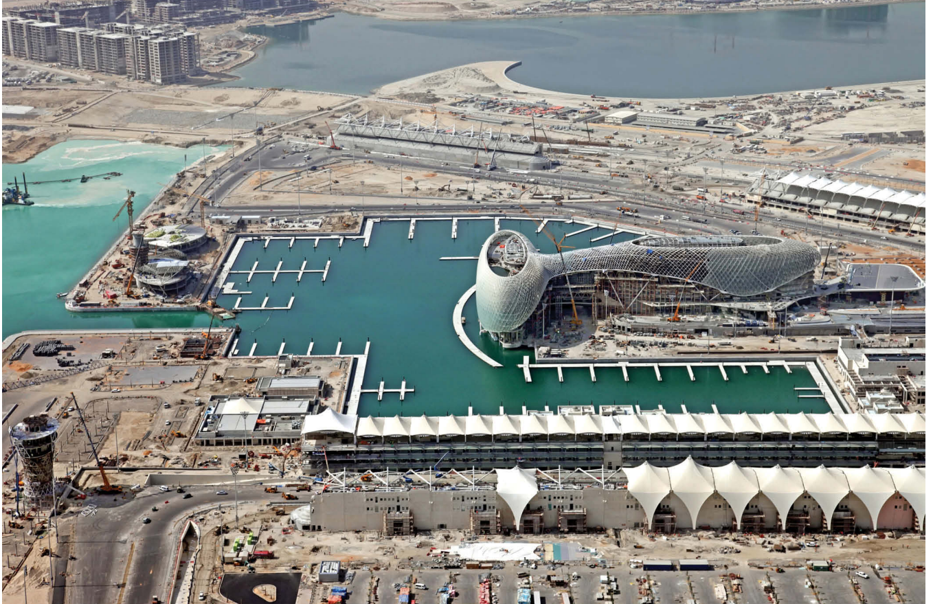
top: Site overview during construction
