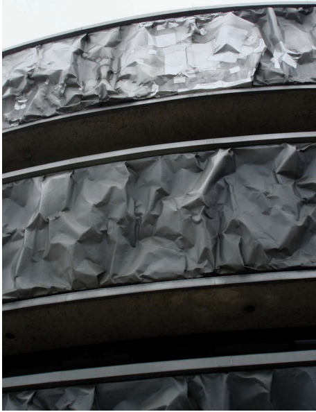
fig. 13 | Because the sheet material is one piece and quite thin, repairs are not easily accomplished.
