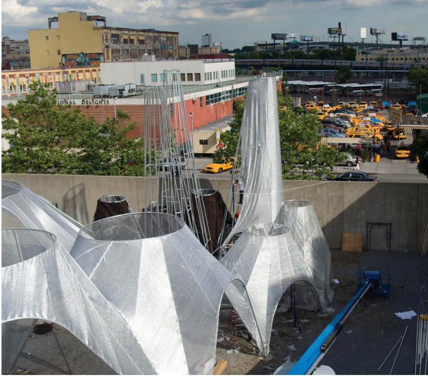
fig. 12 | Construction of aluminum and steel structure and Aluminet, PS1 Afterparty, 2009 (top)
