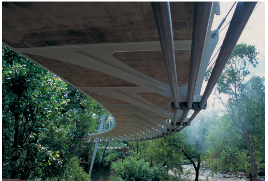
figs. 15–17 | Circular suspension bridge with carefully shaped details, Liberty Bridge, by Miguel Rosales (architect) and SBP, Greenville, South Carolina, 2004
