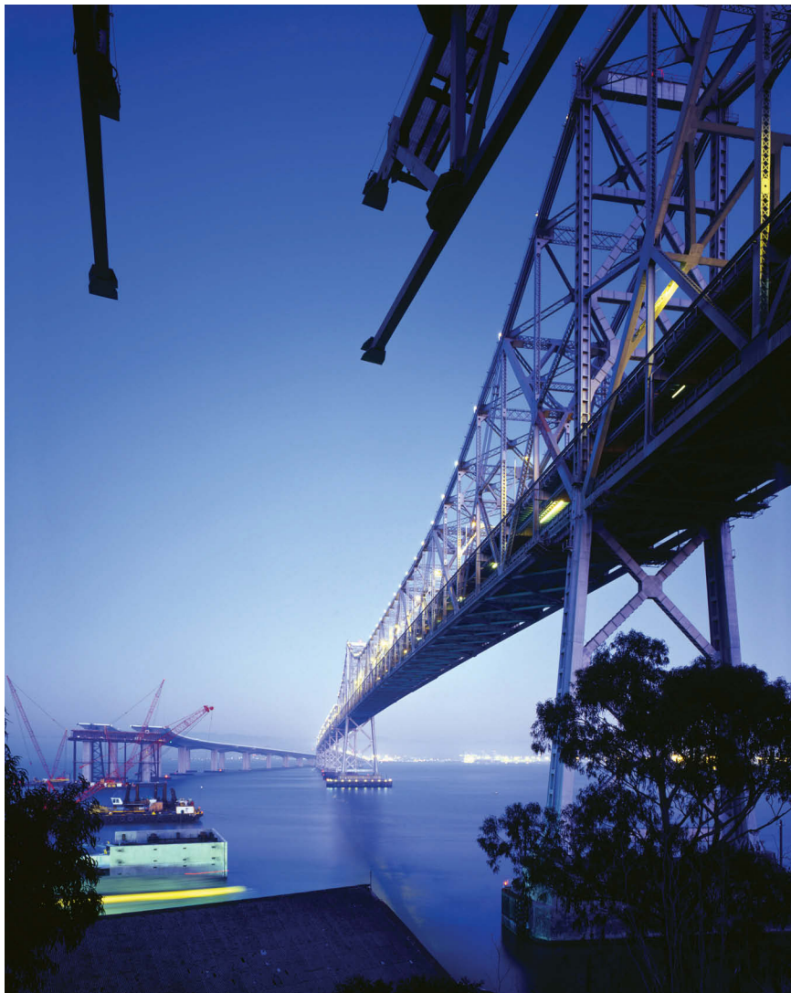
fig. 2 | Twilight image looking east from Yerba Buena Island in San Francisco Bay, showing the temporary support structure and the new span in the background; existing Bay Bridge is shown on right. (top right)
