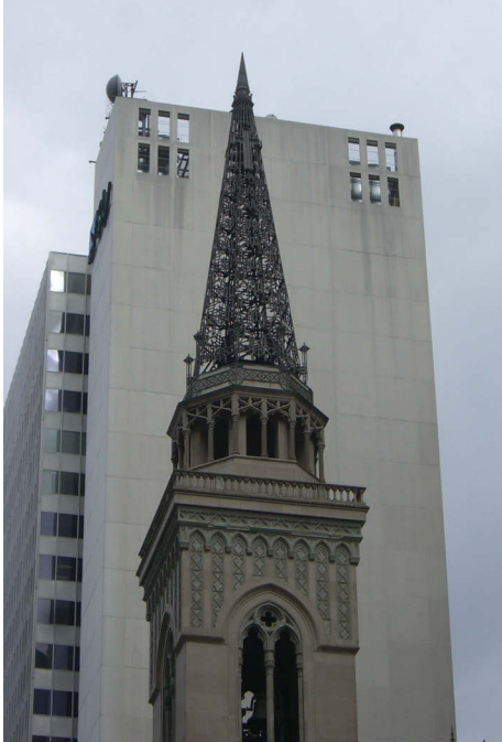
fig. 2 | Cast-aluminum spire, Smithfield United Church, by Henry Hornbostel, Pittsburgh, Pennsylvania, 1926 (left)
