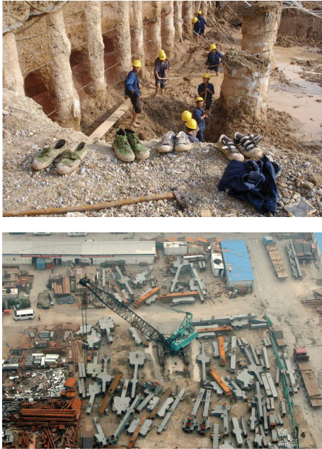
figs. 15–17 | Construction views, CCTV, 2008
