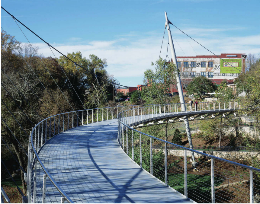
figs. 15–17 | Circular suspension bridge with carefully shaped details, Liberty Bridge, by Miguel Rosales (architect) and SBP, Greenville, South Carolina, 2004
