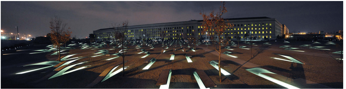
above: View of the Pentagon Memorial, facing east toward the Pentagon, showing the illumination of the units
