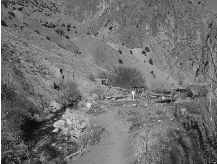
FIGURE 20.13 Available across road into Ort kand.
