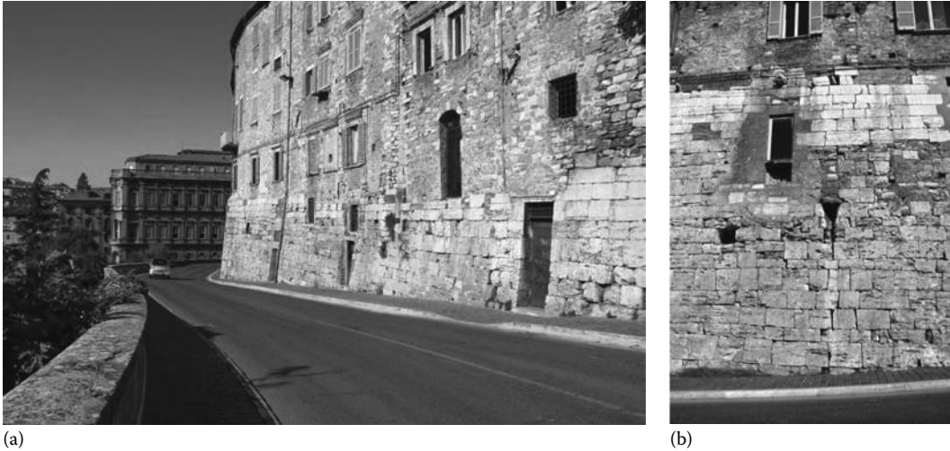
FIGURE 9.10 Perugia, Central Italy: (a) Etruscan walls. The Etruscan walls are those made up with great gray travertine blocks. Medieval walls and houses are on the top of them; the palace in the background was made in the nineteenth century. On the left of the modern road, there are other medieval and modern buildings hiding the Etruscan City. (b) A little drain/sewer out of the Etruscan walls. (Photo courtesy of W. Dragoni.)
