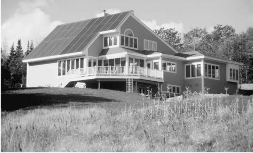
Figure 8.2. Roof integrated PVs and solar thermal panels on a coastal Maine residence (Solar Design Associates, Inc. and DOE/National Renewable Energy Laboratory)
