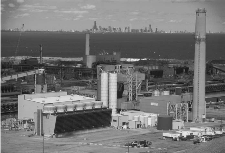
Figure 9.1. Cokenergy – energy recycling plant at Mittal Steel, East Chicago, Indiana
