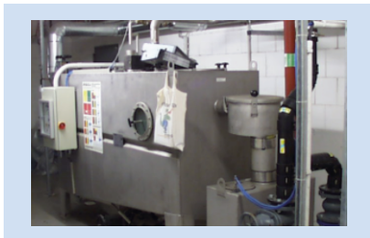
Fig. 3-31 Grease separator
