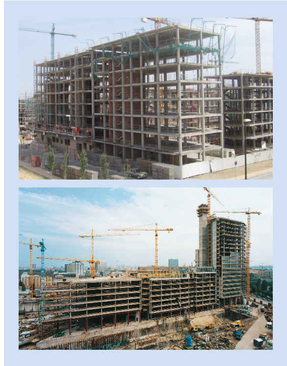
Abb. 3-11 Reinforced steel skeleton construction
