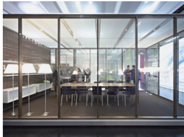
Fig. 3-68 Example light partition wall
