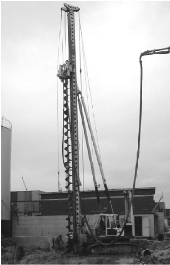
Figure 2.16 Installing CFA piles.
