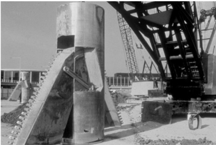
Figure 2.9 Tool for boring underreamed piles.
