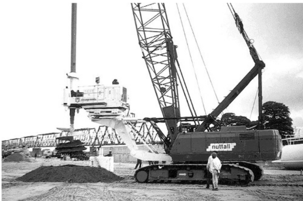
Figure 2.7 Soil removal from auger by spinning off.
