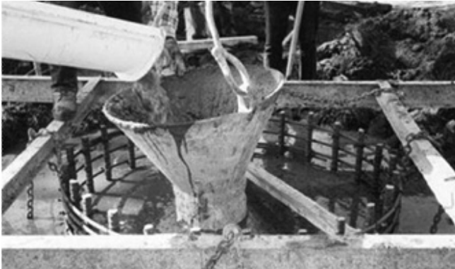
Figure 2.11 Drop chute.
