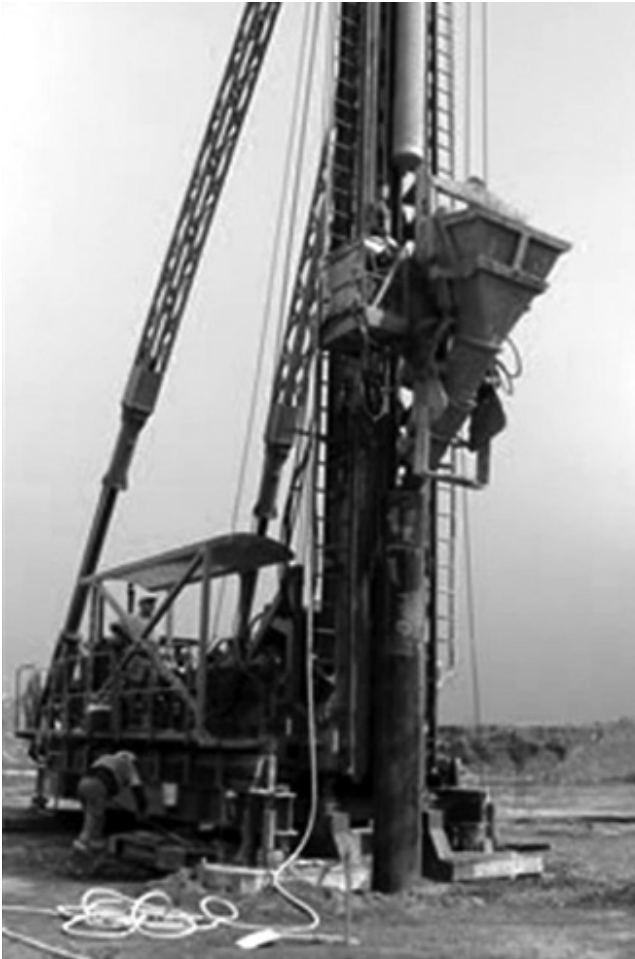
Figure 2.27 Rig for installing Franki piles.
