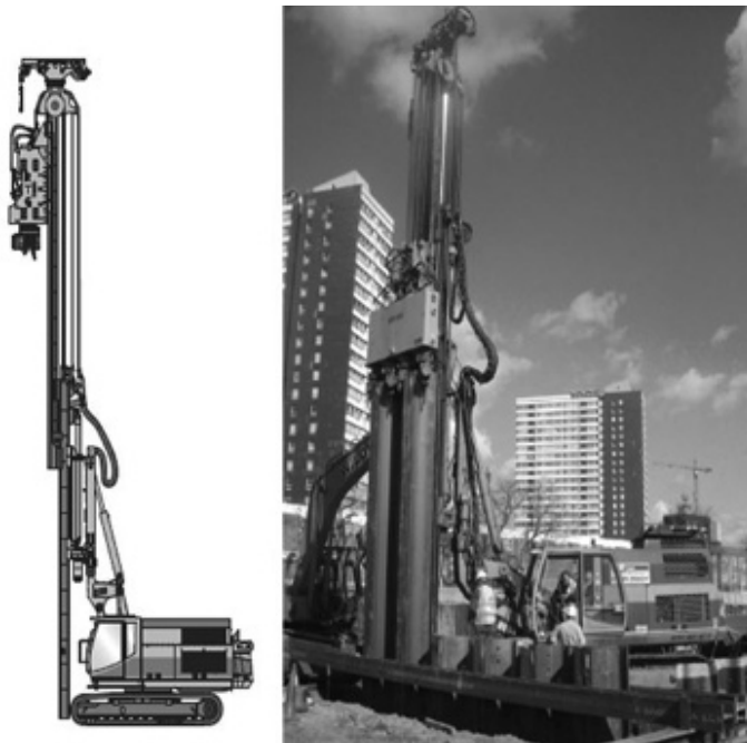
Figure 2.21 Vibratory driving.
