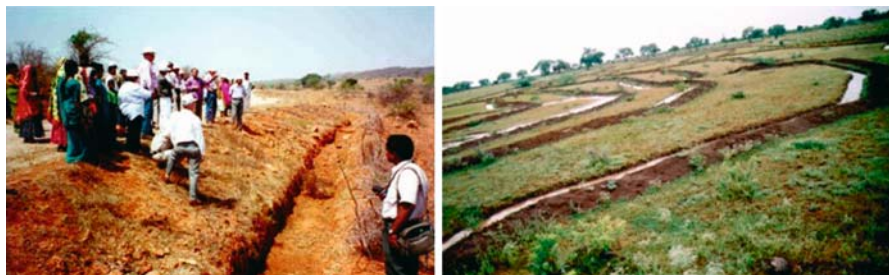
Fig. 15.6 Contour trenching for runoff collection.
