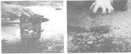
FIG. 5. Coring of asphalt pavement with initial failure.
