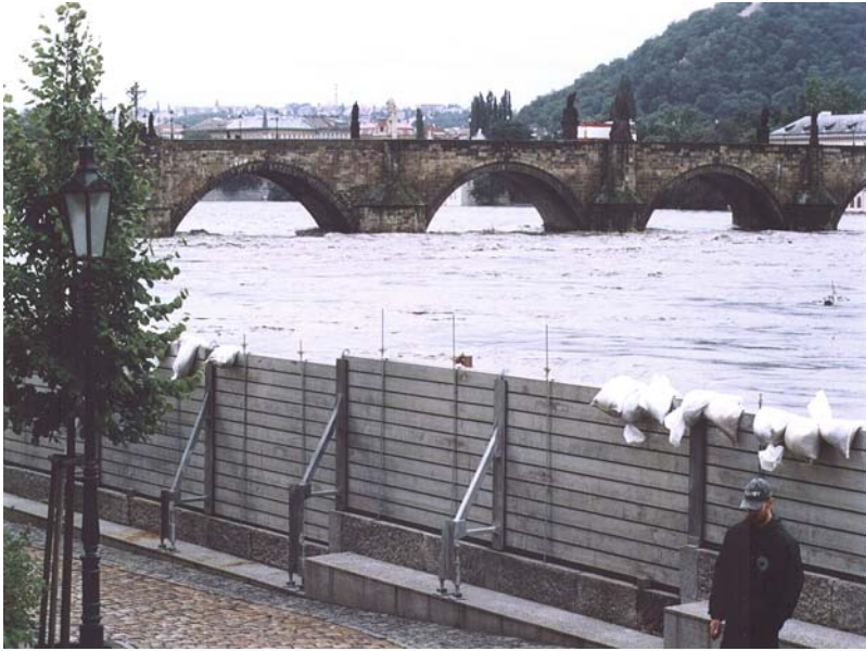
Figure 5. Charles Bridge in Prague on horizon – Forefront- non-permanent flood protection barriers anchored to the pedestrian path with the reinforced foundation platform – the photo was taken during the flood 8/2002 in Prague
