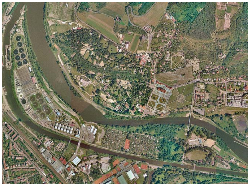
Figure 14. Císařský Island – Central Waste Water Treatment plant (see also Figure 4 13)
