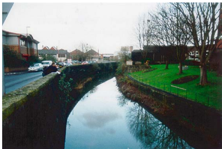
Figure 5. Open channel section of River Frome (downstream of the M32 culvert and immediately upstream of the Frome culvert) illustrating key features of an urban watercourse
