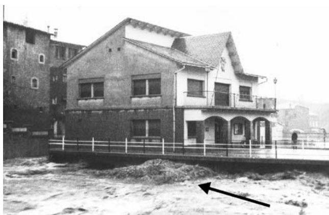
Figure 2. Flow reflection against the bridge pillar – La Pobla de Lillet, Spain, November 1982
