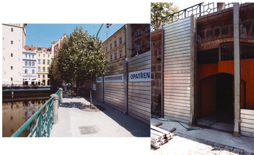
Figure 17. Moveable construction (see also Figure 5) as completed prior flood in 8/2002 – phase 0001 – designed by Hydroprojekt a.s. – total cost 90M CZK (3M Euro)
