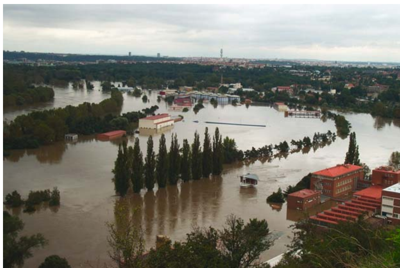
Figure 4. Flooded Water Research Institute T.G.M. (building on the left) and the Central Waste Water Treatment Plant (within the area laced by the line of trees)- downstream edge of Prague
