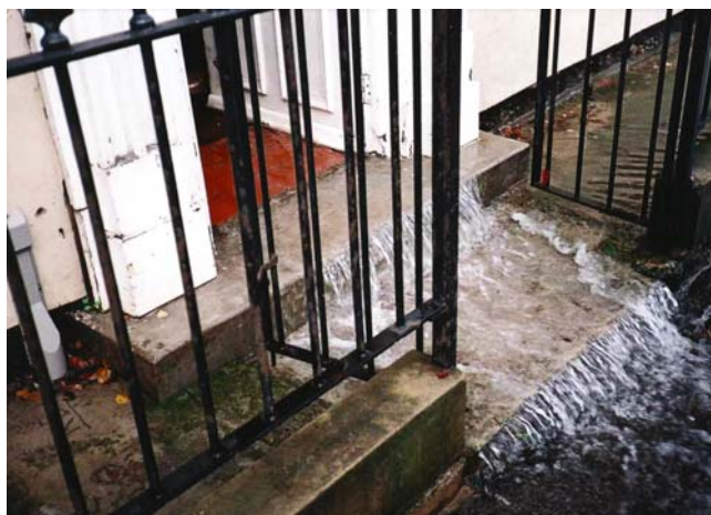
Figure 3. Opening doors lets floodwater flow in or out (Malton, England, 2000)
