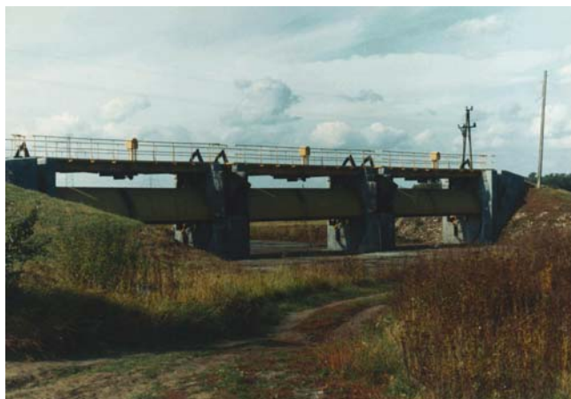
Figure 11. The inlet sluice structure for the polder near Trestno close to Wrocław
