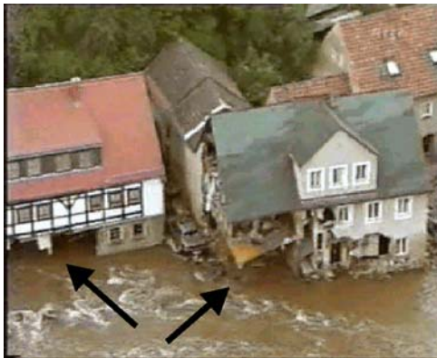
Figure 3. Sharp angle of a house cut by the flood wave in Weisenstein, Germany, during the summer of 2002
