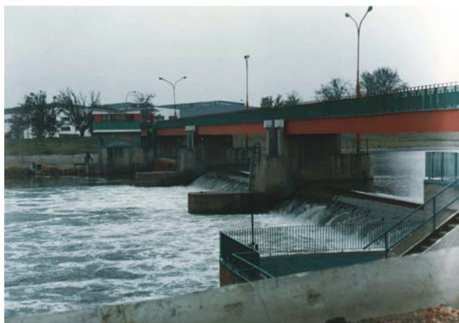
Figure 10. The moveable gate structure at Opatowice upstream of the town of Wroclaw
