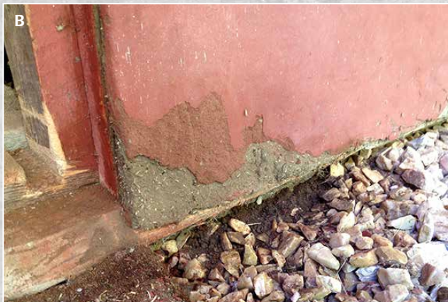
A: broken vinyl siding; B: clay plaster damage; C: clay plaster repair. CREDIT: CHRIS MAGWOOD
