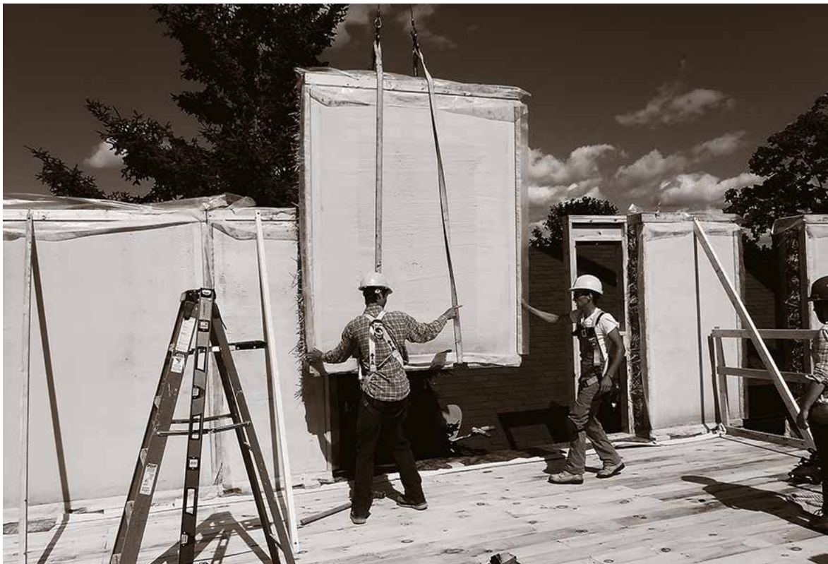
SIP panel guided into place and fastened.
