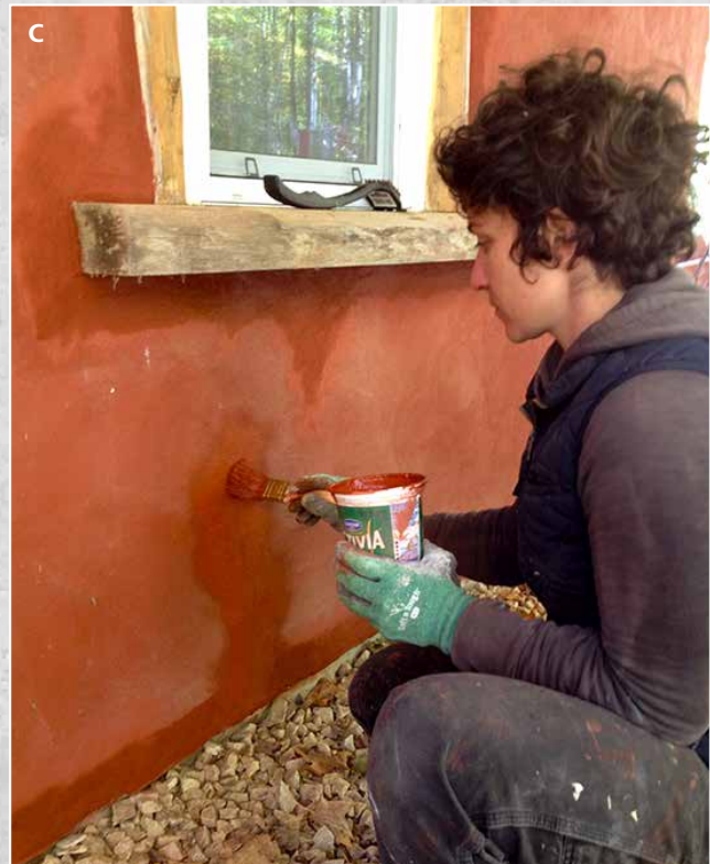
A: broken vinyl siding; B: clay plaster damage; C: clay plaster repair. CREDIT: CHRIS MAGWOOD
