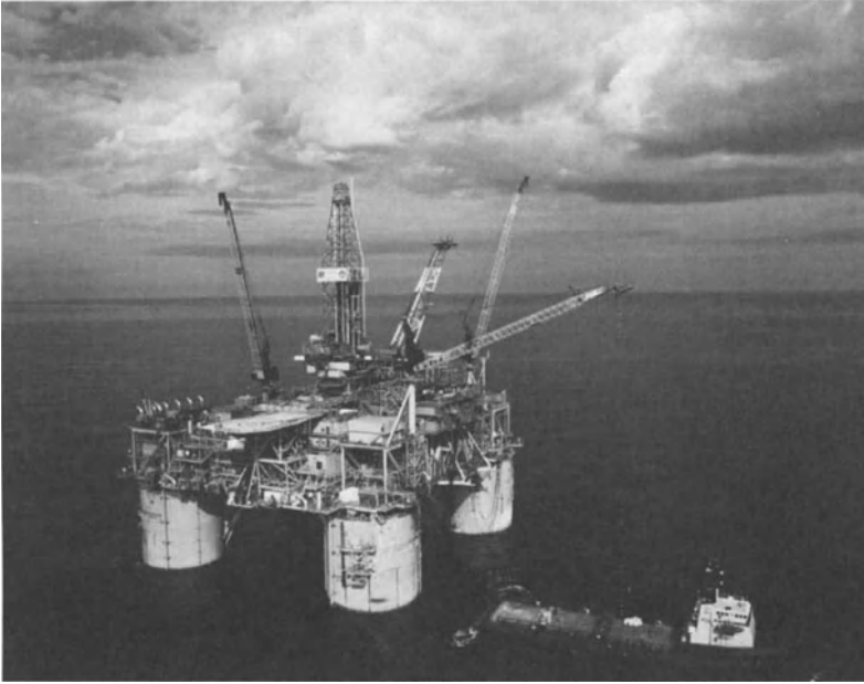
Figure 1.2. The Ursa TLP (Courtesy of Shell Exploration and Production Company)
