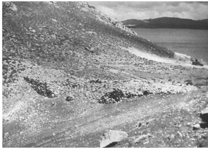
Figure 3. Ruins of the southern Kesis Gölü dam, the oldest gravity dam in the world (Photo G.Garbrecht).
