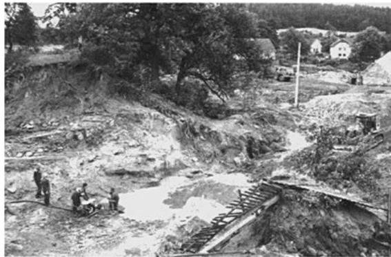
Photo 1. Dam Metelsky—gash with old wooden outlet.
