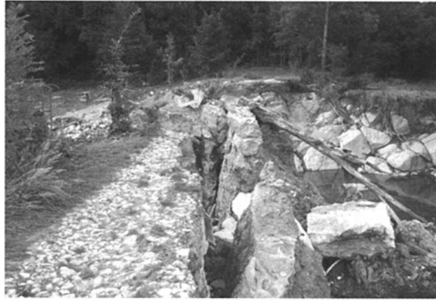
Photo 5. Dam Podhajsky—old clay-cement jet injection sealing wall.
