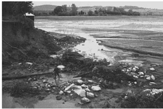
Photo 1. Dam Metelsky—gash with old wooden outlet.
