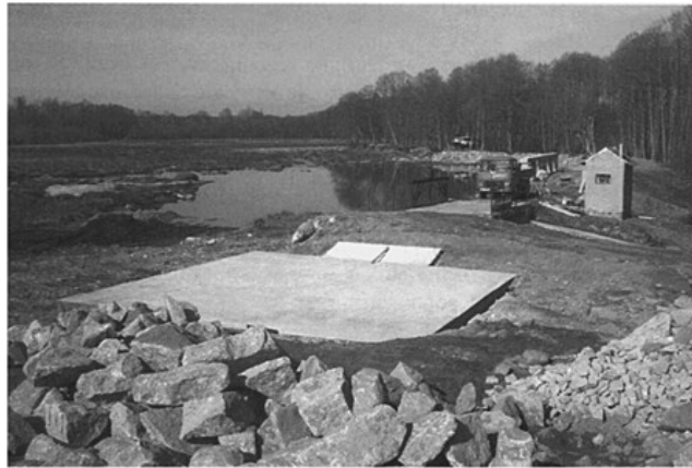
Photo 9. Dam Dolejsi—new additional unprotected spillway.
