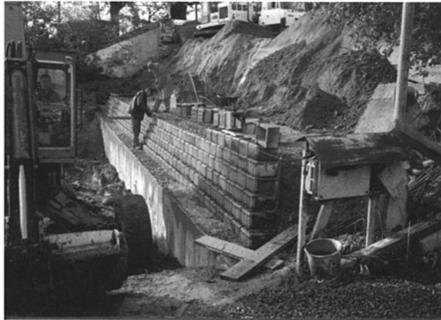
Photo 6. Dam Horejsi—retaining wall from the reinforced soils.
