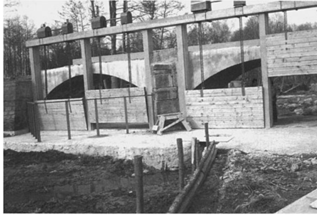
Photo 8. Dam Dolejsi—new spillway (4 pcs)—without middle pillar.
