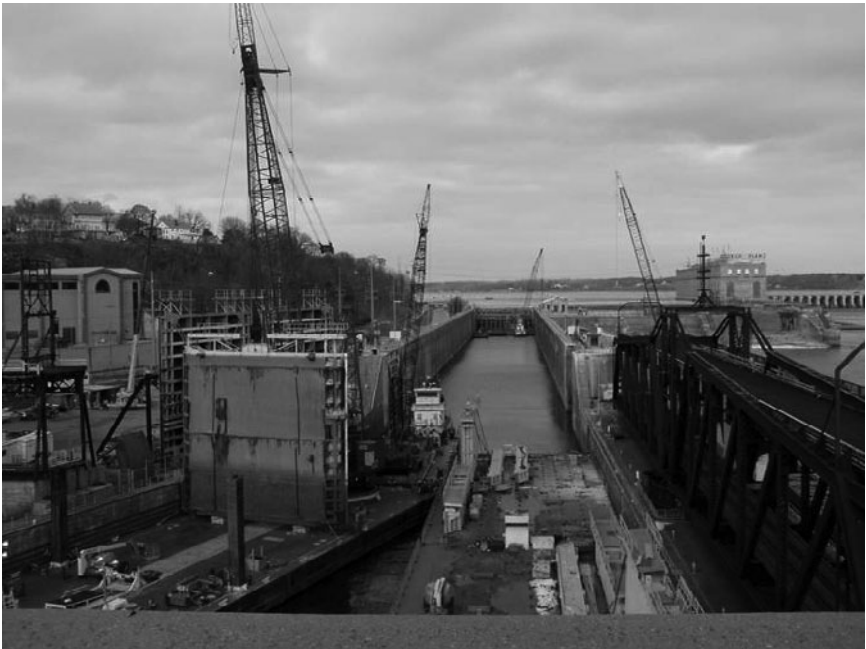
FIGURE 8-2. Lock 19 Major Maintenance Work. Courtesy of U.S. Army Corps of Engineers.
