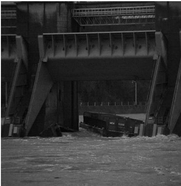
FIGURE 8-3. Barge Caught in Dam by High Flows. Courtesy of U.S. Army Corps of Engineers.
