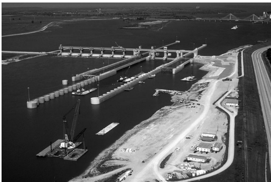
FIGURE 5-4. Melvin Price Lock and Dam, Mississippi River near Alton, Illinois. 24-Foot Lift. Courtesy of U.S. Army Corps of Engineers.
