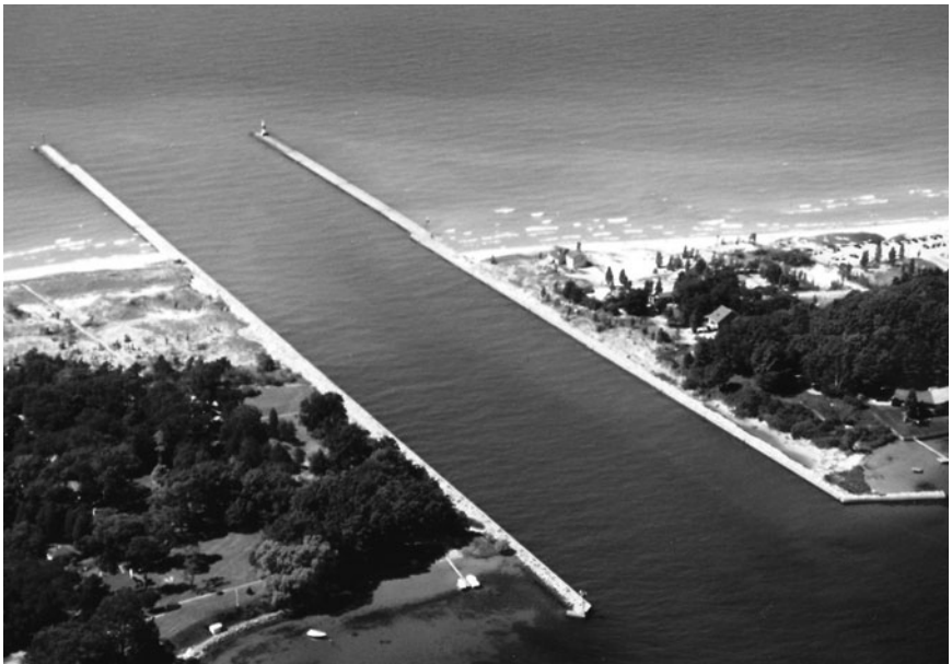
FIGURE 5-10. Jetties, Portage Lake Harbor, Onkama, Michigan. Courtesy of U.S. Army Corps of Engineers.
