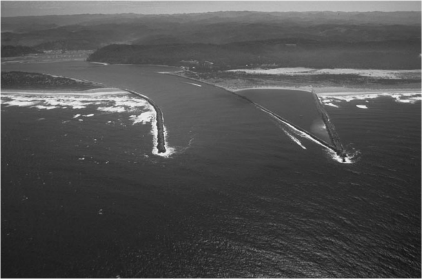
FIGURE 5-11. Jetties, Entrance to Umpqua River, Oregon. Courtesy of U.S. Army Corps of Engineers.
