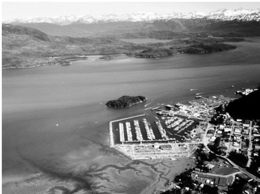
FIGURE 5-6. Small Boat Harbor, Cordova, Alaska. Courtesy of U.S. Army Corps of Engineers.
