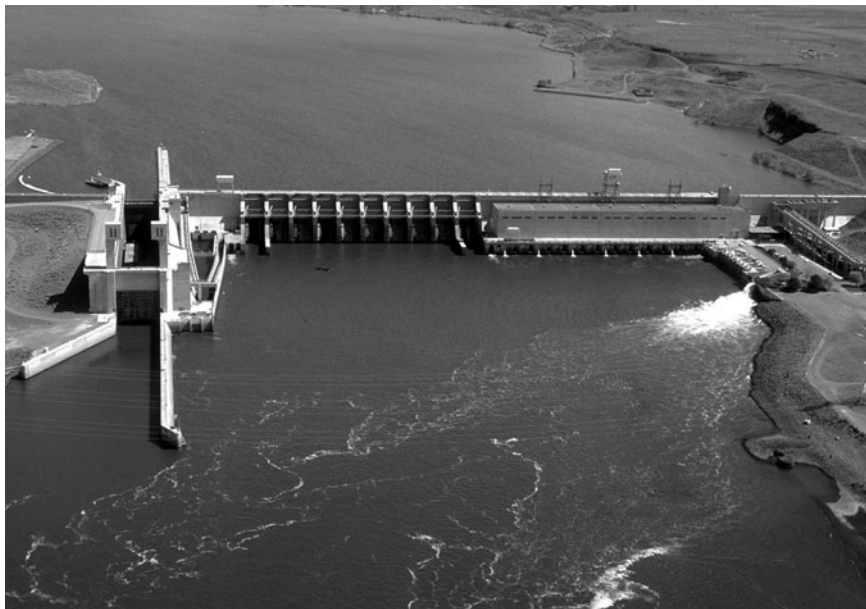
FIGURE 5-3. Ice Harbor Lock and Dam, Snake River, Washington. Lift 100 Feet. Courtesy of U.S. Army Corps of Engineers.
