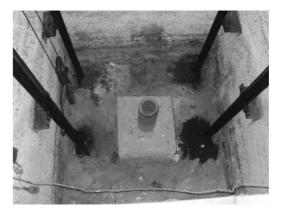
Photograph 3. Electric wiring present in the elevator shaft.
