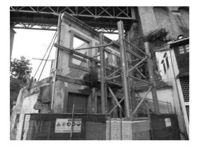
Figure 2. Facade of building with materials containment.
