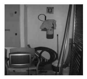
Photograph 1. Access to the machine room being obstructed by objects.
