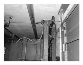
Photograph 2. Folded ironwork from the elevator's cabin door.
