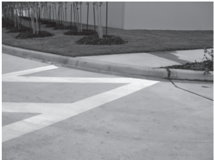
Figure 2.6b: This accessible route does not have a curb ramp where it crosses a curb.
