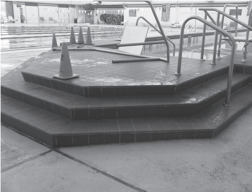
Figure 4.36: A pool with steps up to it requires at least one means of access.
