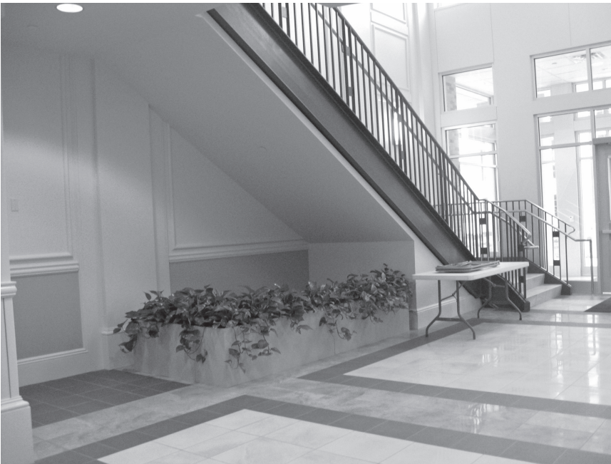
Figure 10.23: An open stair would require a way to stop a person from hitting their head with the treads behind the stair. In this case, a planter was used to enhance the space as well as to shield the hazard.
