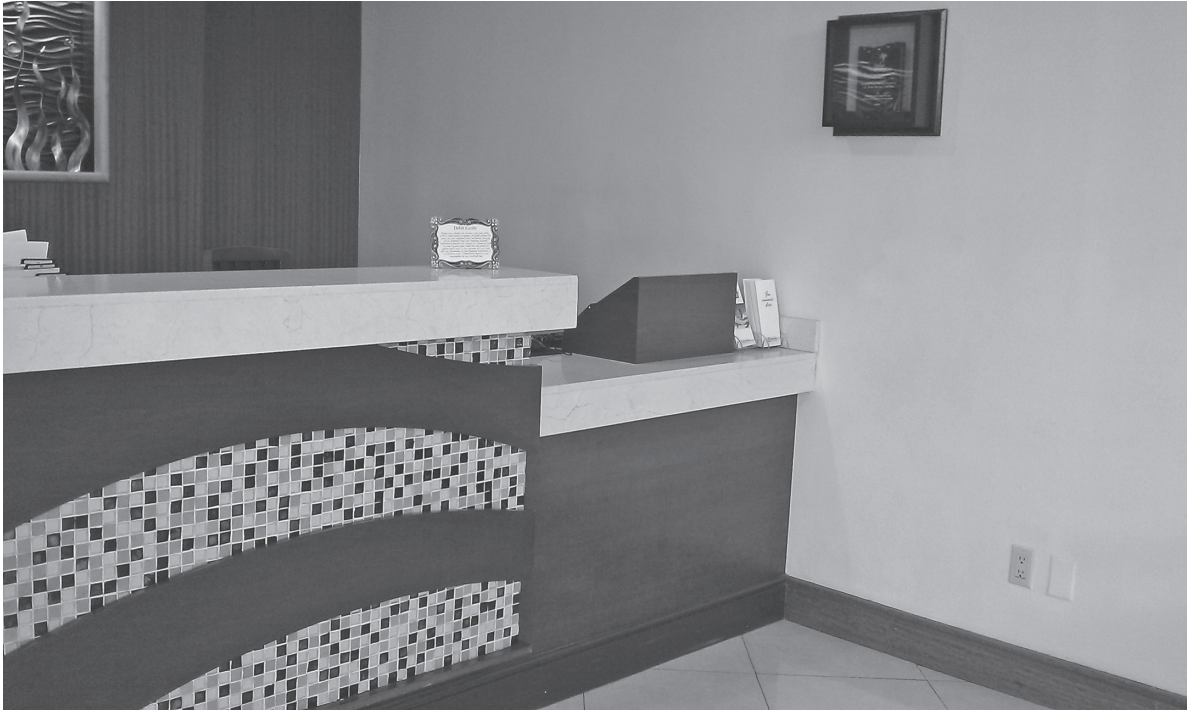
Figure 5.2: Registration counter—avoid cluttering the accessible counter. Sundry Shop/Retail
