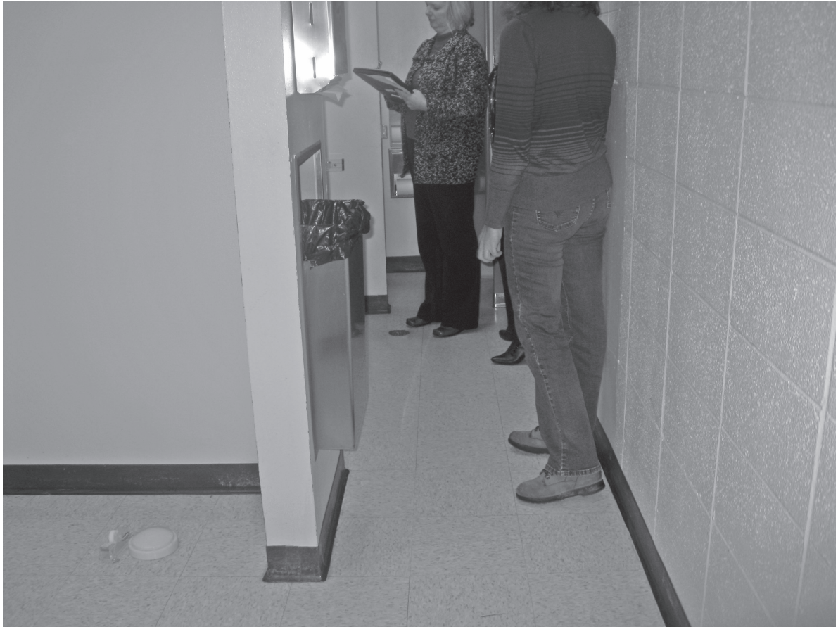
Figure 8.4: This new paper towel dispenser reduced the accessible route width to the toilet compartment.
