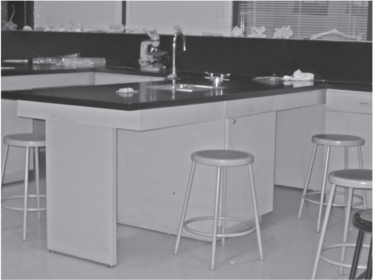
Figure 3.6: Lab counters must have a knee space and be at an accessible height.
