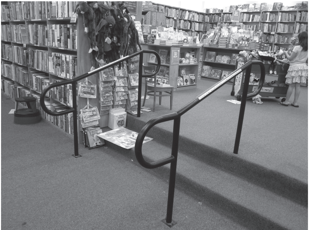
Figure 2.10: If there are any level changes within the store, an accessible route should connect each level. These steps cannot be the only access to the upper level of the store.
