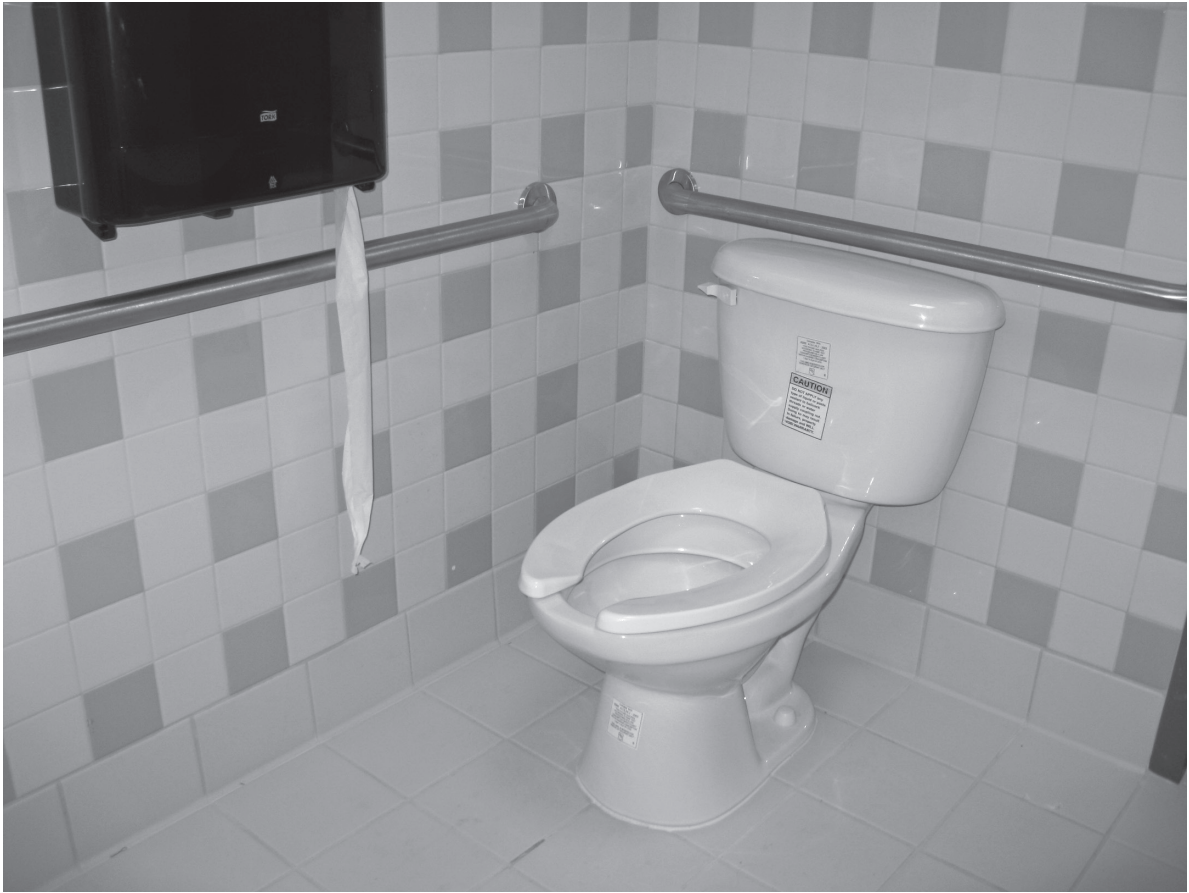
Figure 3.23: Water closets for children should not be a tank type if the grab bar heights for children will be used. The distance between the tank and the grab bar should be 12 inches minimum in order to allow for gripping.
