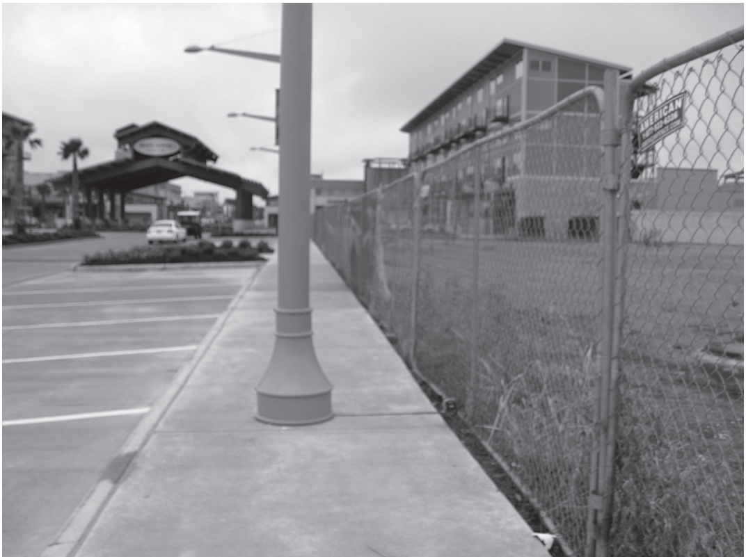
Figure 2.45: A lamp post is impeding access along the accessible route.
