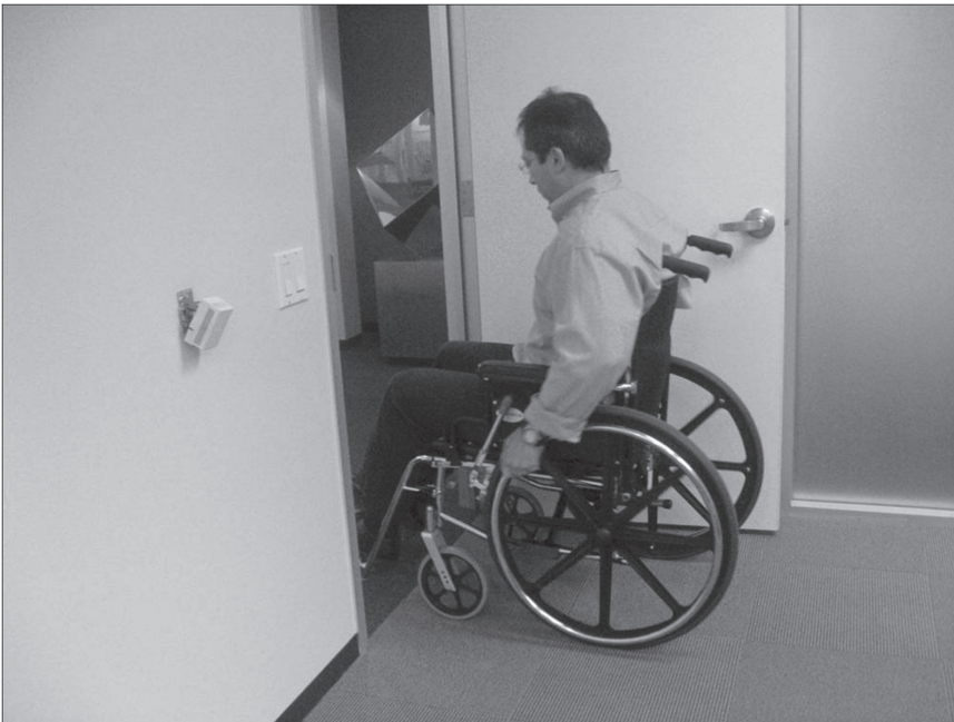
Figure 10.11: A universal design for a doorway will not take less than 5 seconds to close.
