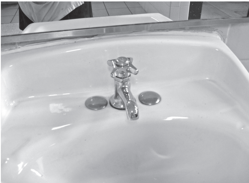
Figure 1.8: An accessible operable part should not require tight grasping or twisting of the wrist to use.
