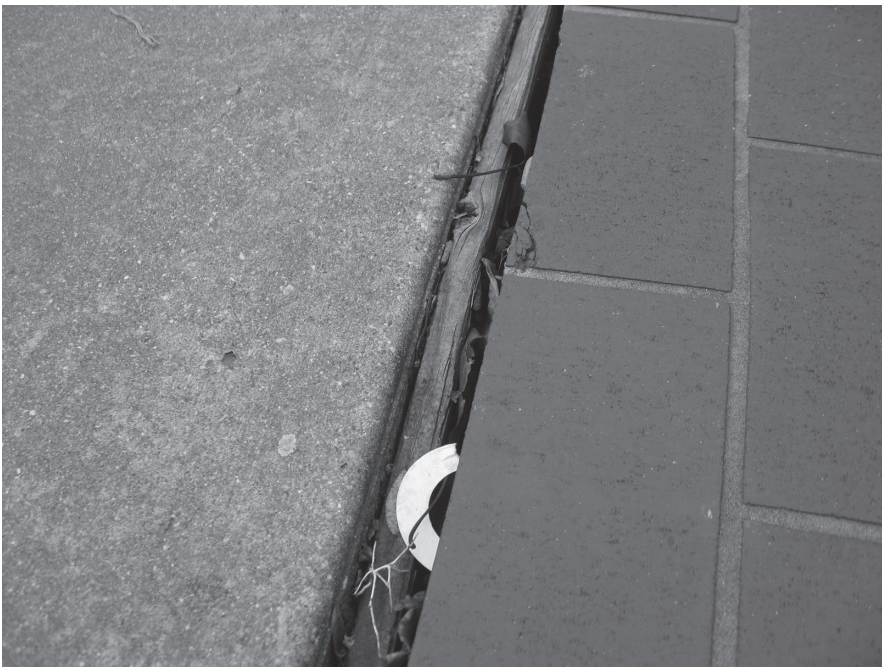
Figure 2.8: Gaps along the path of travel to the mall must be avoided. The wood expansion joint located at this sidewalk decayed away and created a gap wider than \frac{1}{2} inch.
