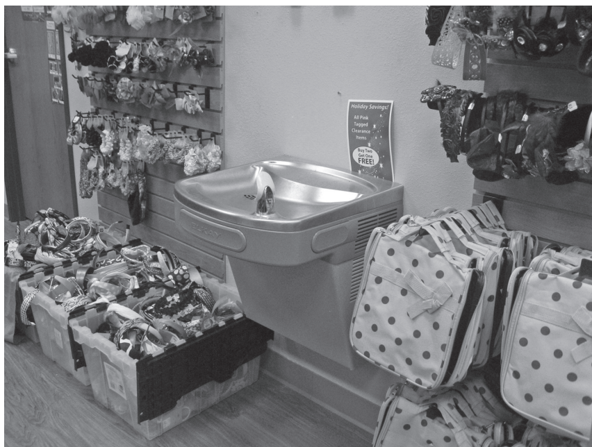
Figure 2.12b: Drinking fountains should have proper clearances.
