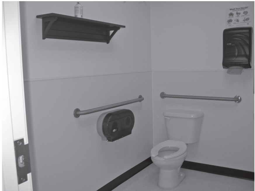
Figure 3.10: Shelving at restrooms must also be at an accessible reach range.
