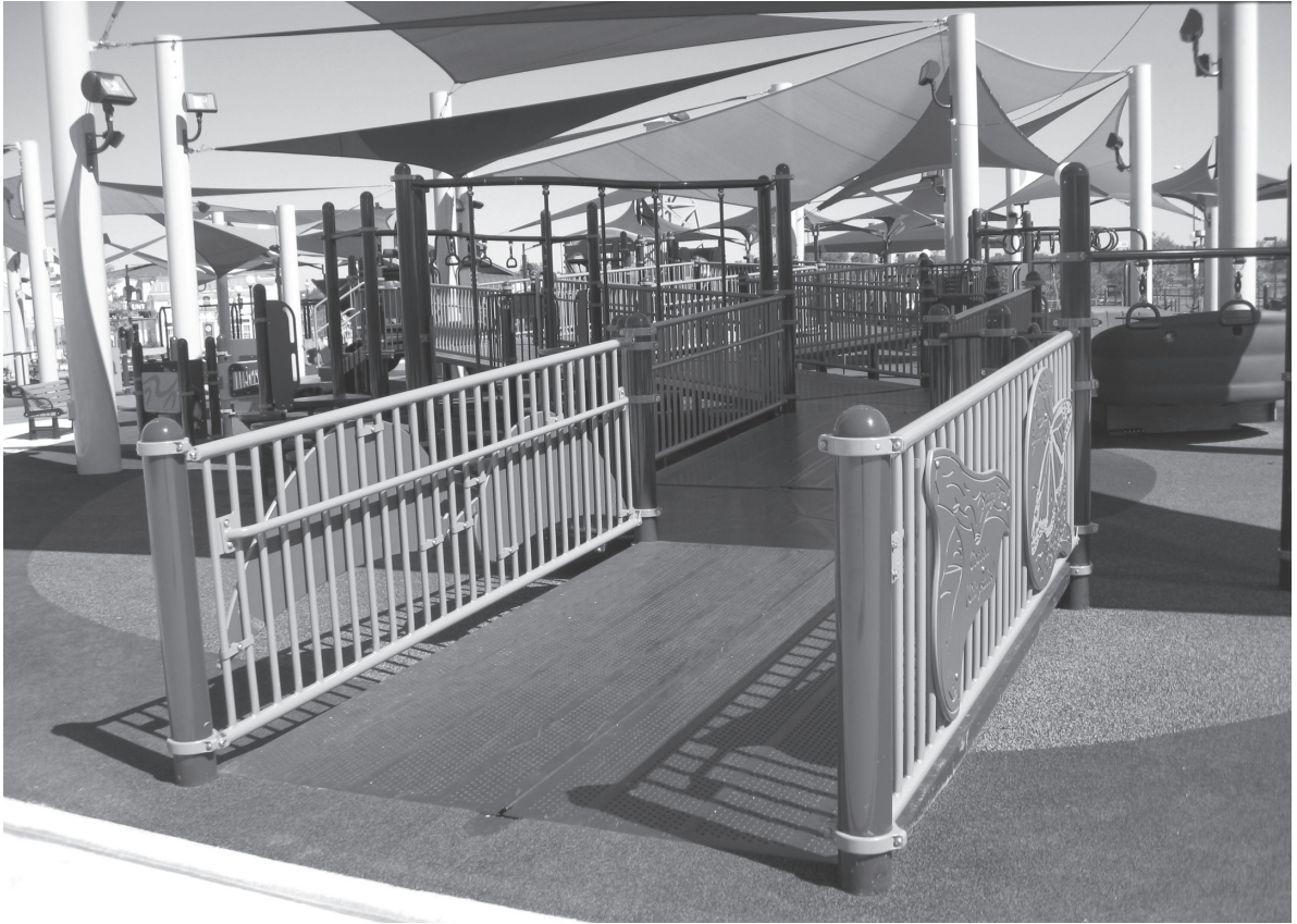
Figure 7.11: Ramps connecting ground-level play components to elevated components is one method of connection.
