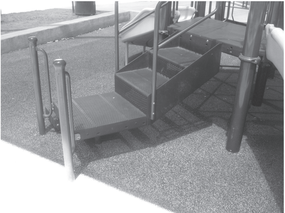
Figure 7.13b: Transfer steps allow children with different abilities to use play components together.
