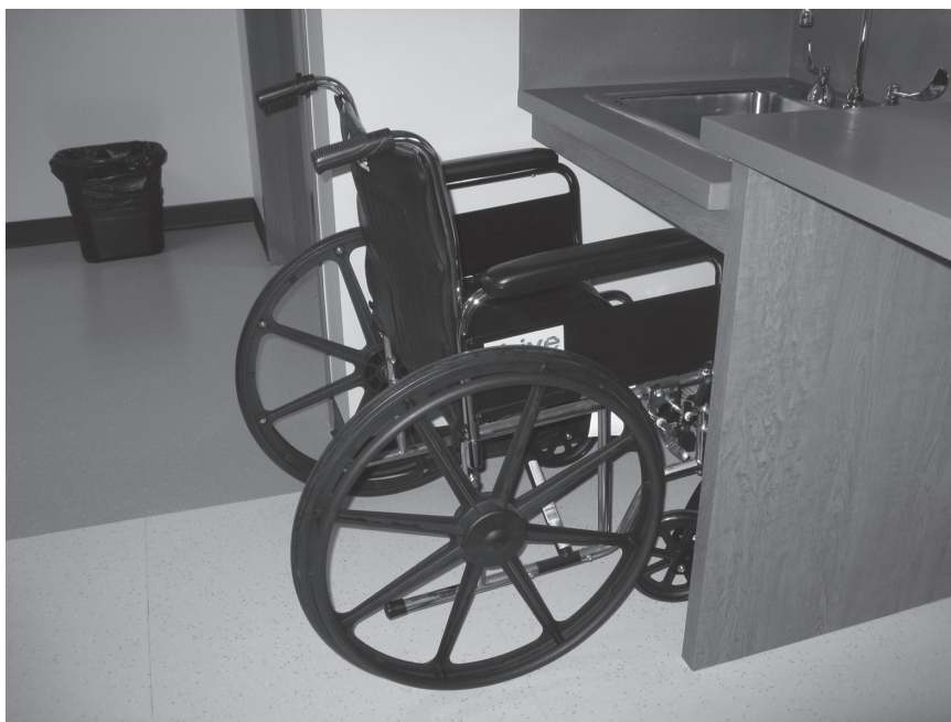
Figure 4.20: A knee clearance for wheelchairs should be provided at classroom sinks.
