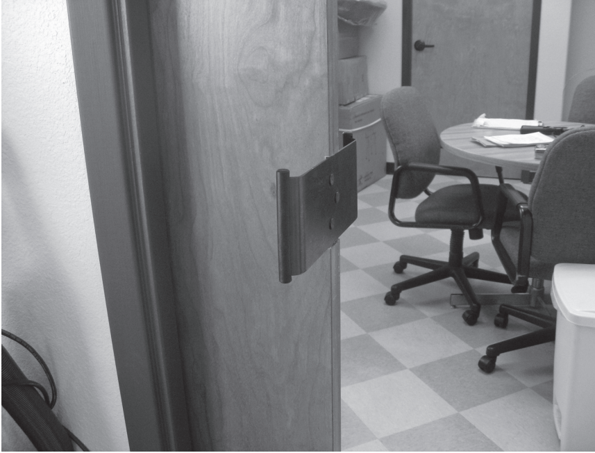
Figure 2.48a: Pocket doors should have hardware that, once the door is open, will allow the 32-inch minimum clearance to enter.
