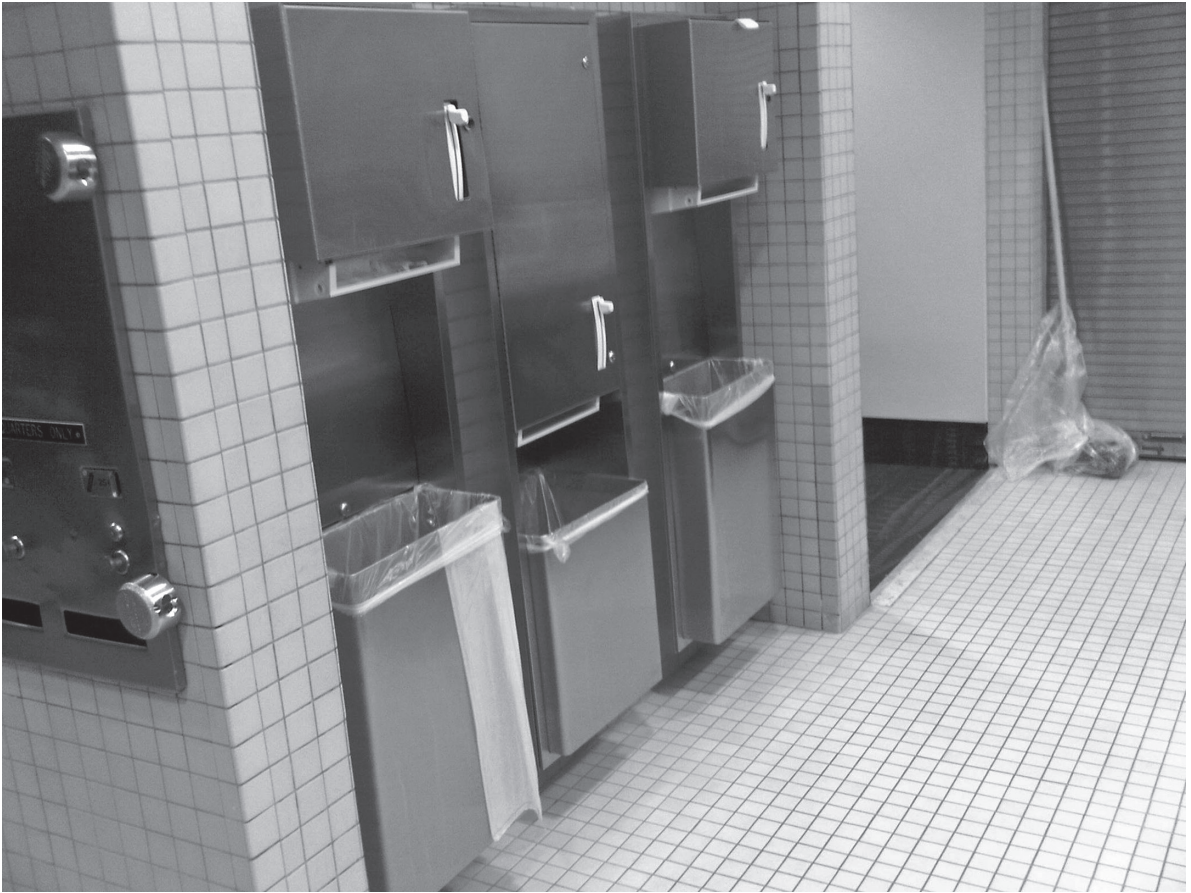
Figure 2.50: Using recessed fixtures ensures that no protruding objects will be found along the circulation path of the restroom.
