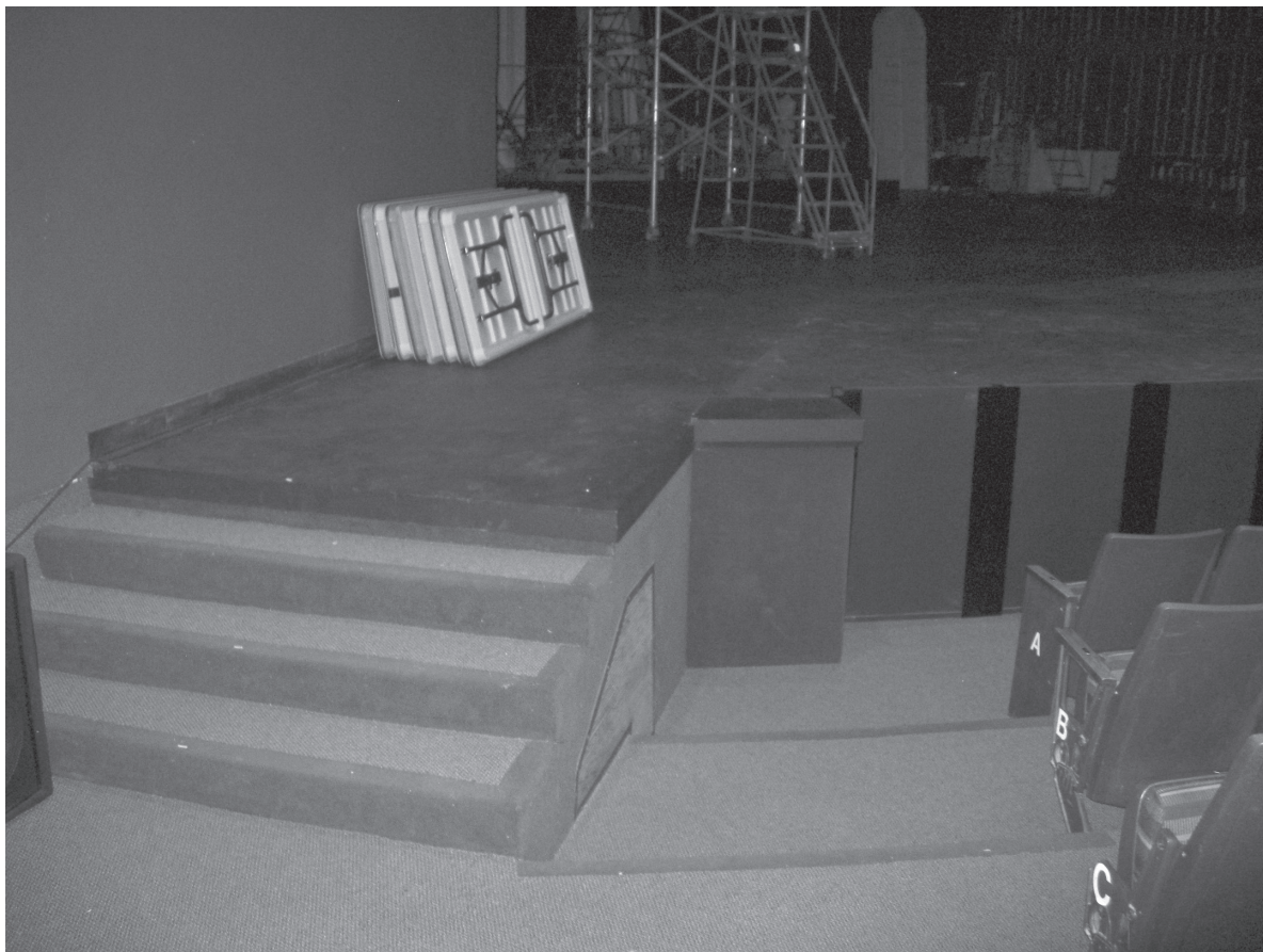
Figure 4.15: Access to the stage from the audience seats is required if there are steps or other means to access the stage from the spectator seats.
