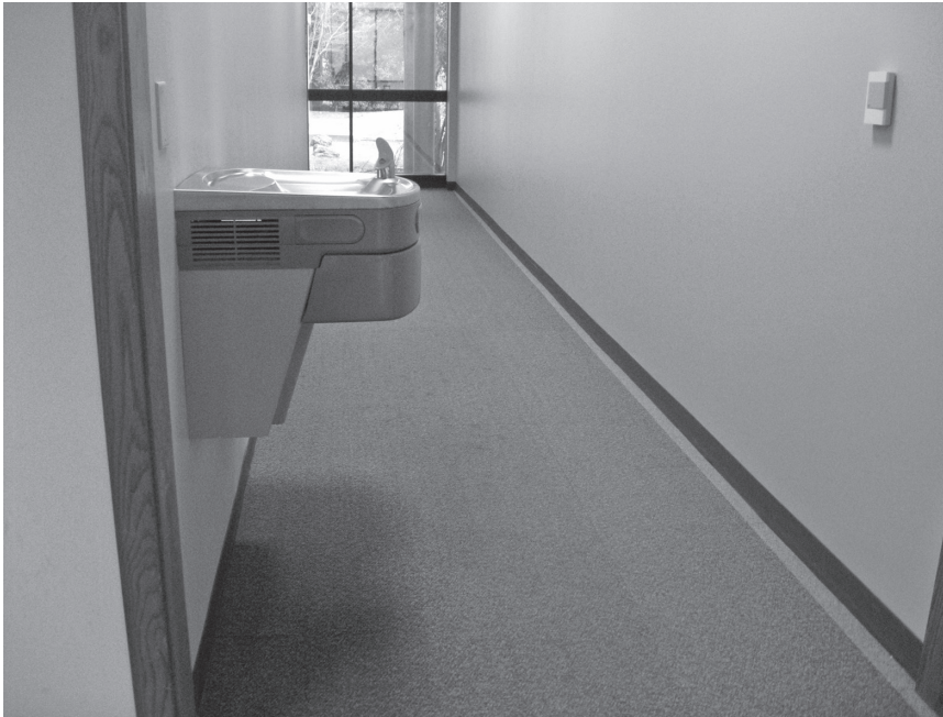
Figure 2.23: The common path of travel should be free from hazards for the visually impaired. This drinking fountain might be a hazard to a blind person if either of the units is mounted higher than 27 inches above the ground measured to the bottom of the fountain.
