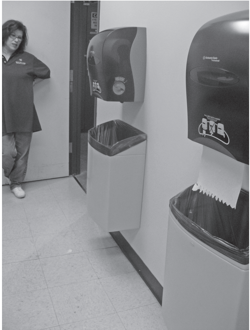
Figure 8.2: This existing paper towel dispenser was a protruding object until the permanent waste paper basket was installed below it.
