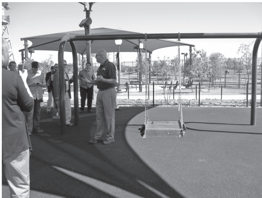
Figure 7.15a, 7.15b: Swings for disabled children can take many forms. This one allows a wheelchair to be strapped inside in order for the child to swing while he is in his wheelchair.
