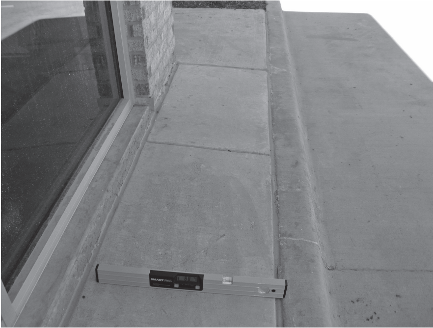
Figure 2.7: An accessible route should be a minimum of 36 inches wide. The sidewalk shown in the photograph is only 24 inches wide.
