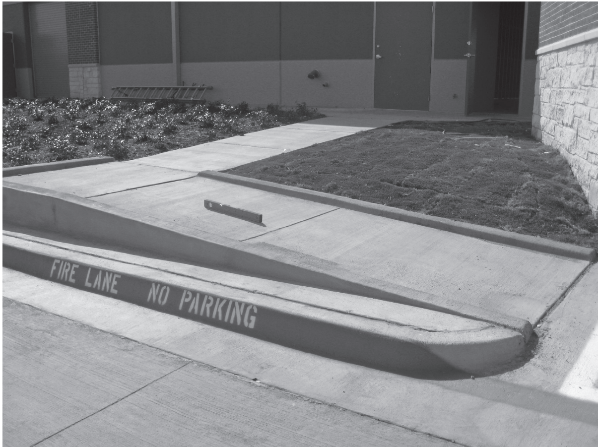
Figure 10.33: A curb ramp is a good example of an element which minimizes physical effort. It is easier to use than lifting objects over the curb.
