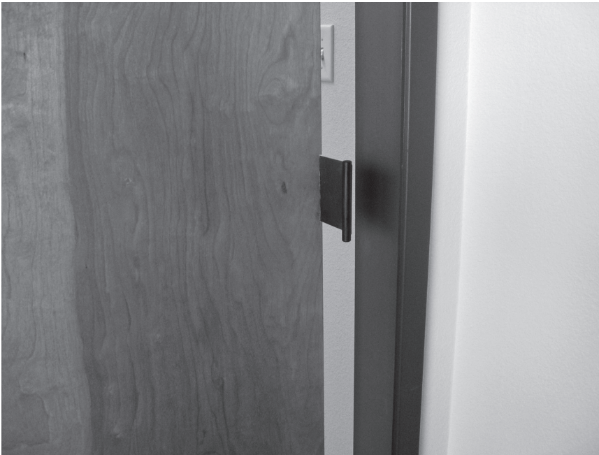
Figure 2.48b: Pocket door hardware should be able to be used without tight grasping and twisting of the wrist.
