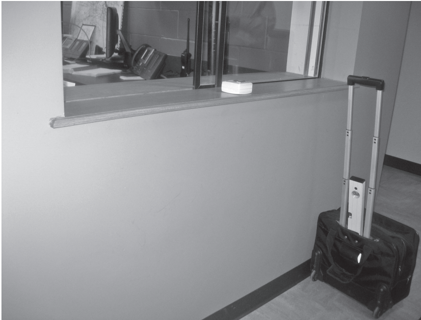
Figure 2.46c: A reception desk or transaction window should be mounted no higher than 36" a.f.f.
