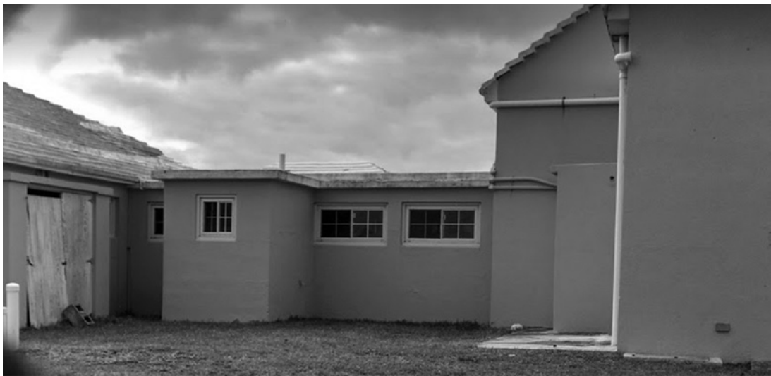
Figure 19-1 Photo of Water Collection System in Bermuda. Water is piped from roof tiles to cistern below building.
