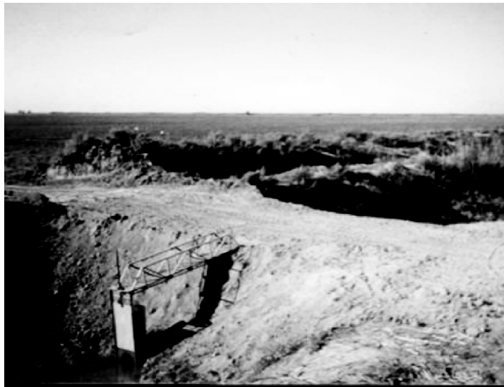
Figure 2. Sluice-regulator on collecting and drainage net.
