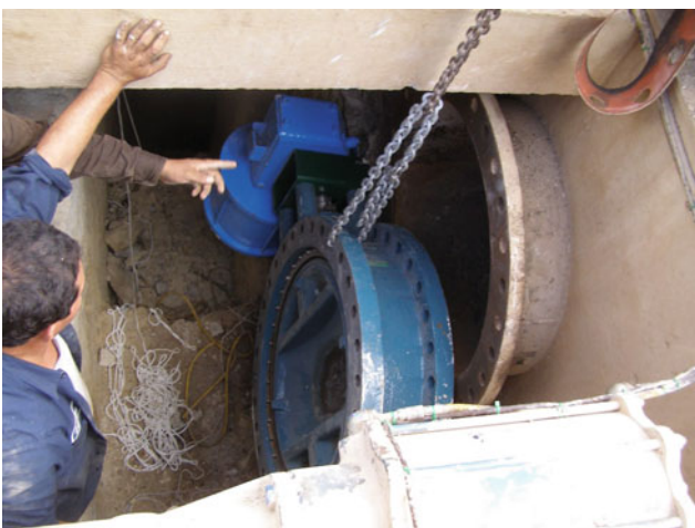
Fig. 8 Installation of second valve (automated) on Antioch BMP
