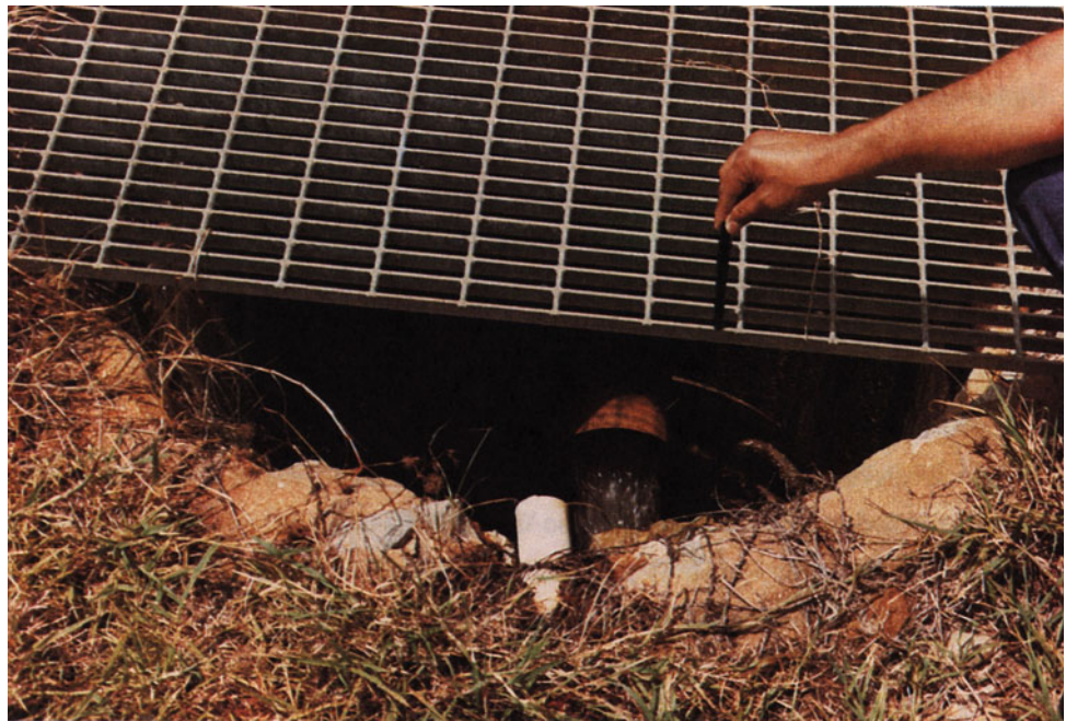
Fig. 6 Industrial wastewater disposal into a reinforced sinkhole at the RCA del Caribe Superfund Site, Barcenoneta, P.R. The reinforced sinkhole was classed as an injection well and the wastewater disposal was operated under an approved permit
