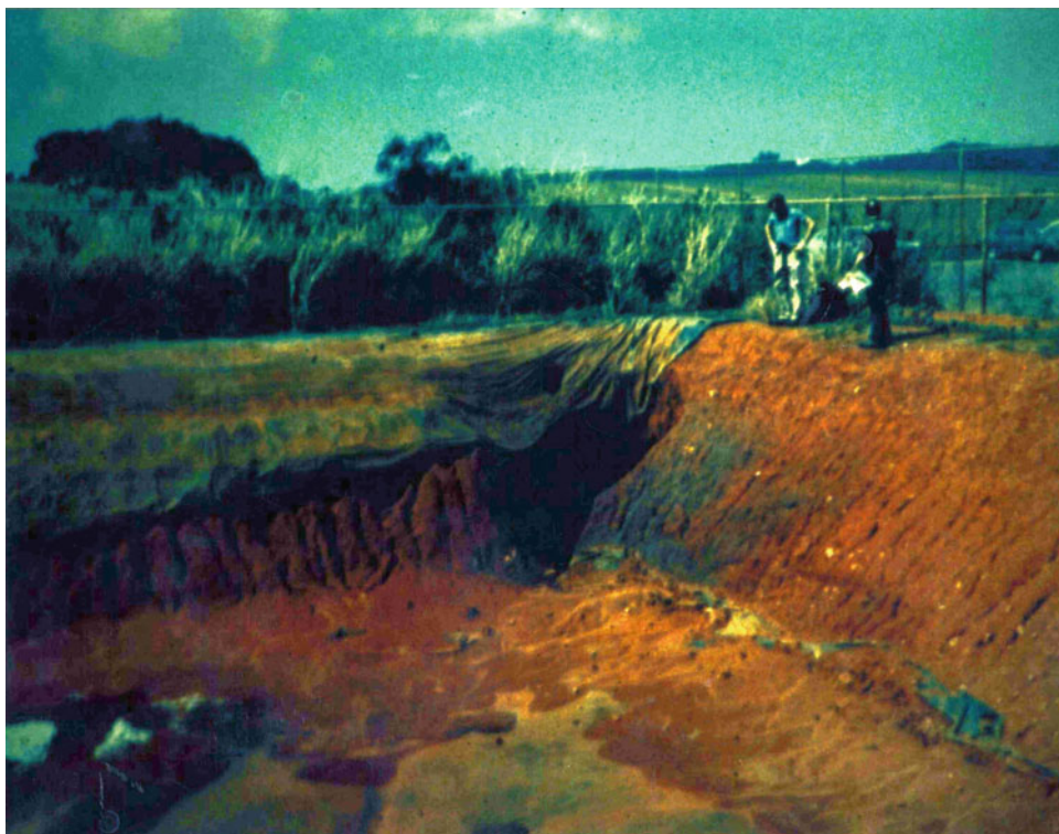
Fig. 9 Lined liquid hazardous waste surface impoundment operated at the RCA del Caribe Superfund Site, Barceloneta, P.R that was breached by a large sinkhole. All the liquid waste was rapidly flushed underground
