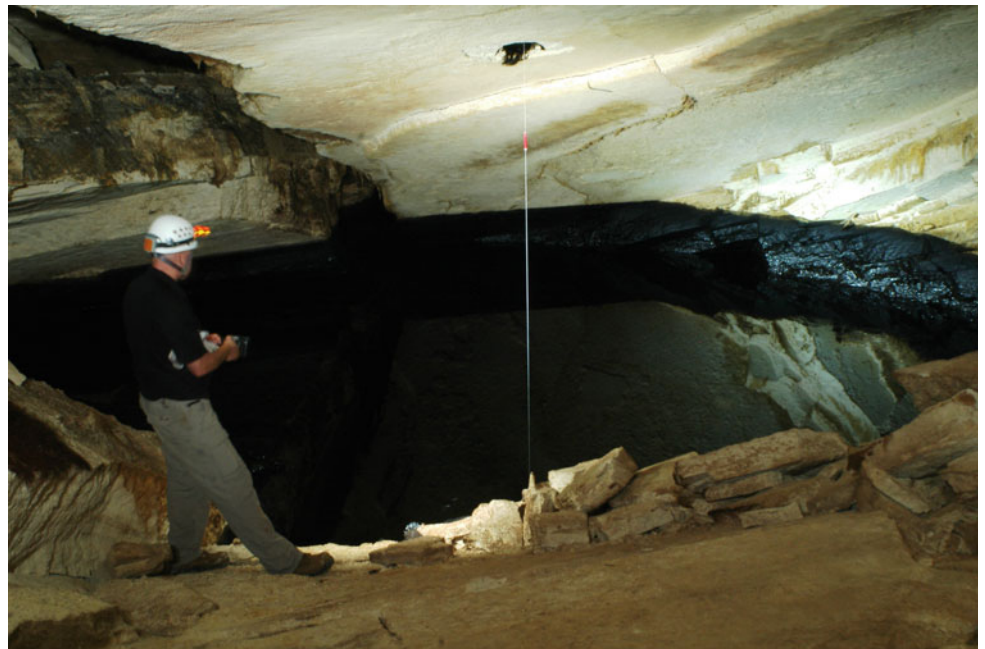
Fig. 8 Oil pool and light stick lowered down boring at west end of the cave
