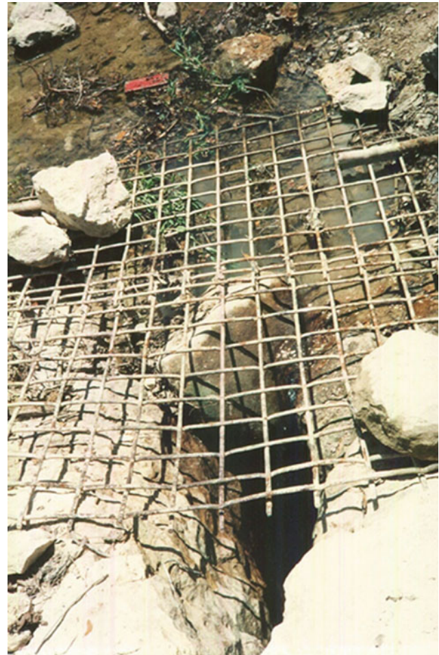
Fig. 2 Photograph ca. 1996 showing recharge and the entrance to Antioch Cave before the BMP was constructed. The debris over the entrance and also sedimentation within the cave decrease the amount of recharge entering the cave (Photograph from Fieseler 1998)
