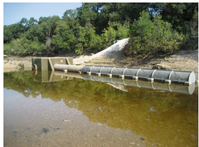
Fig. 9 View of Antioch BMP following upgrade completion. View looking upstream
