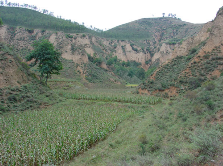
Fig. 5.4 Part of the cascade of check-dam reservoirs in the western main valley in Yangjuangou
