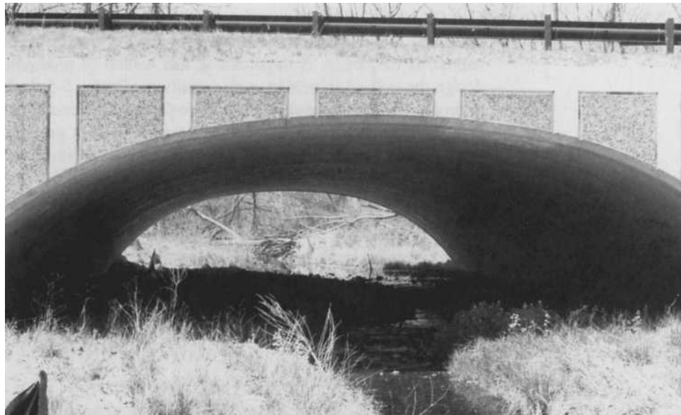
FIGURE 13-6 AN ARCH CULVERT SPANNING A SENSITIVE STREAM AND WETLAND AREA.
