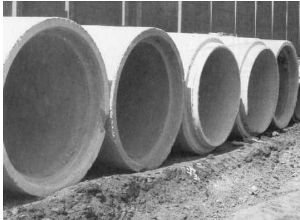
FIGURE 12-3 TYPICAL STORM SEWER PIPE SECTIONS.
