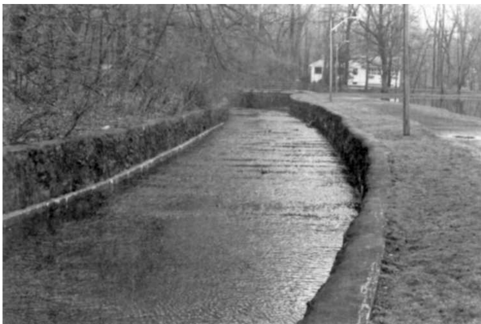
FIGURE 6-2 OPEN CHANNELS ARE OFTEN USED TO CONVEY STREAM FLOW IN DEVELOPED AREAS. THIS CHANNEL HAS A RECTANGULAR SHAPE WITH STONE SIDES.
