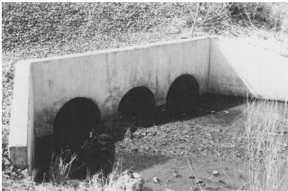
FIGURE 13-2 TYPICAL THREE-BARREL PIPE CULVERT.
