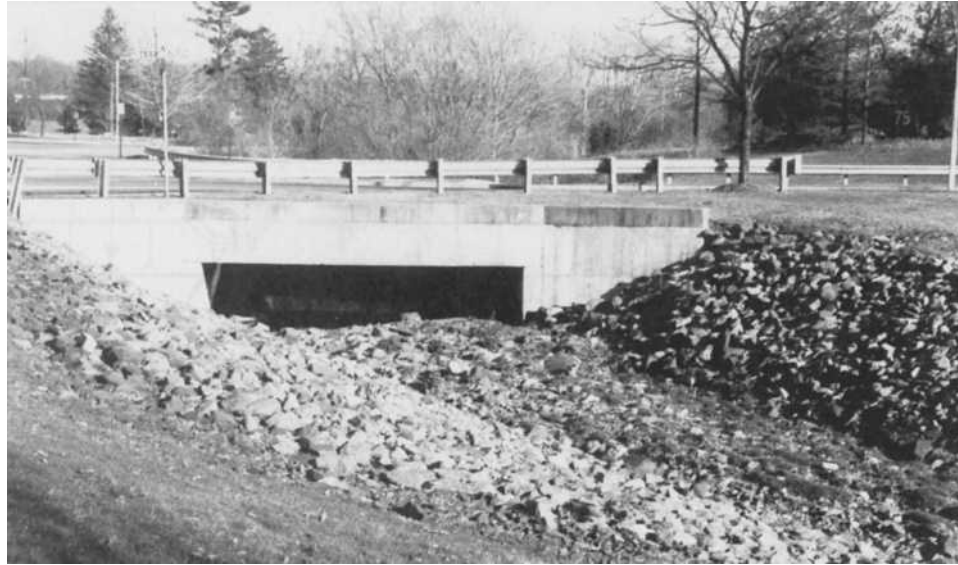
FIGURE 13-4 EXTENSIVE RIPRAP PROTECTS THE TRAPEZOIDAL CHANNEL ON THE DOWNSTREAM SIDE OF THIS NEW CONCRETE BOX CULVERT.
