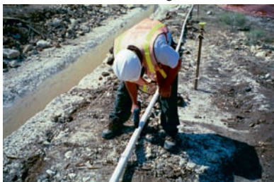
Photo 5 Injection pipe construction
