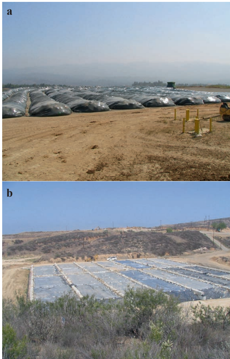
Figure 11.5. Full-scale ex situ soil bioremediation in (a) Ag-Bag ® and (b) concrete containment cells (reprinted from Evans et al., 2008).
