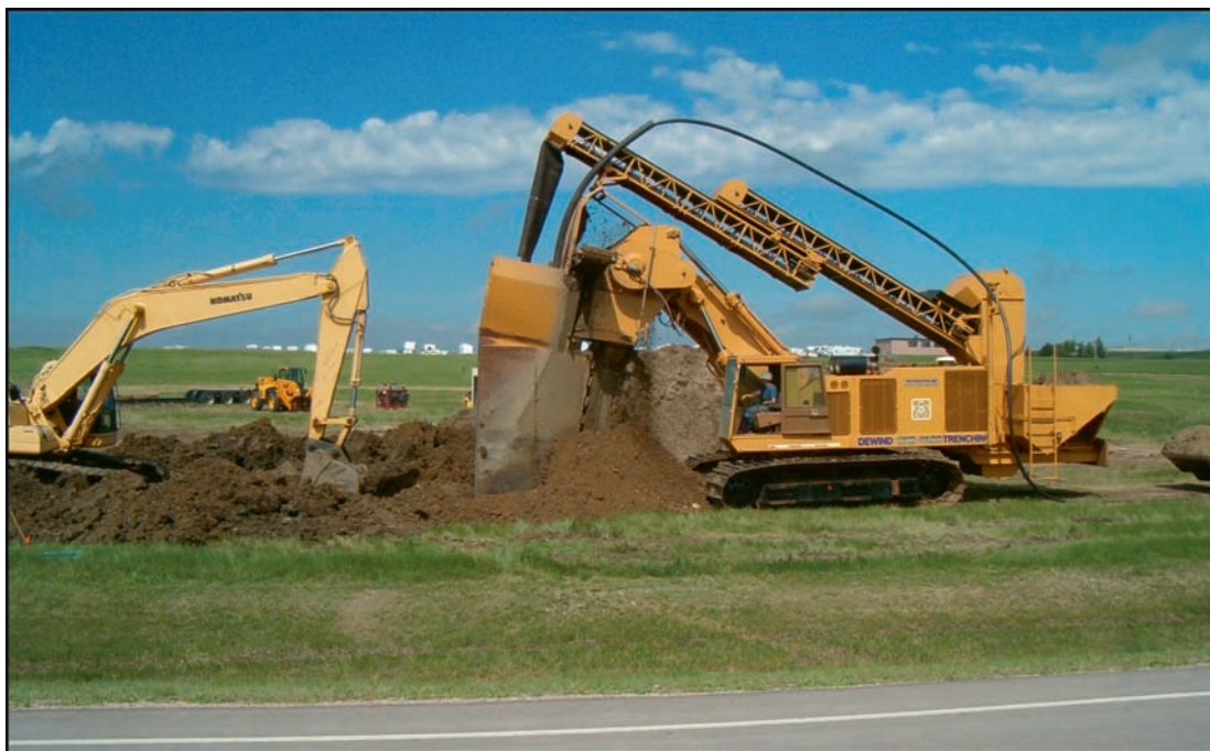
Figure 9.2. Continuous one-pass trencher in operation at Ellsworth Air Force Base, South Dakota (from AFCEE, 2008)
