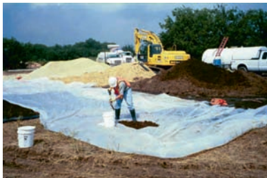
Photo 3 Biowall media before placement
