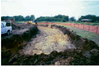
Photo 1 Biowall site preparation
