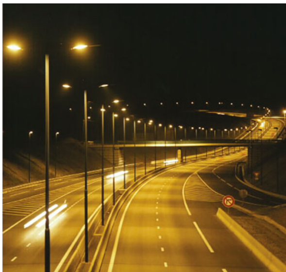
Fig. 13.7 Example of good visual guidance obtained by the alignment of the luminaires
