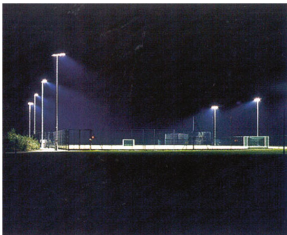
Fig. 18.3 Limiting light pollution by the use of luminaires with sharp, narrow beams aimed downwards towards the field from medium-height poles
