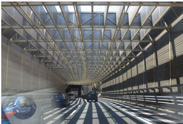
Fig. 22.3 Open non-sunlight daylight screens
