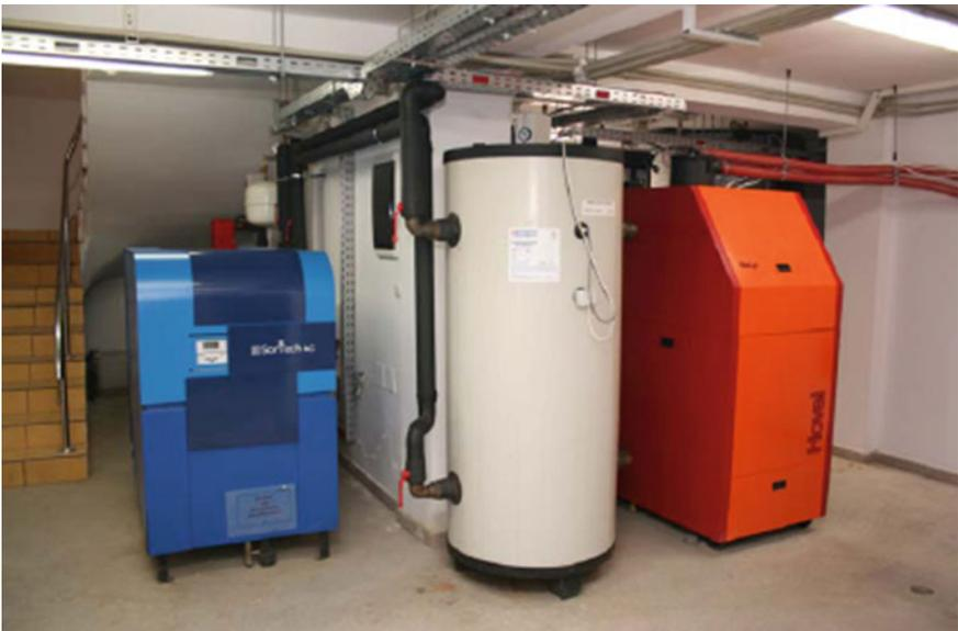
**Picture 1** Adsorption chiller and pellets boiler
