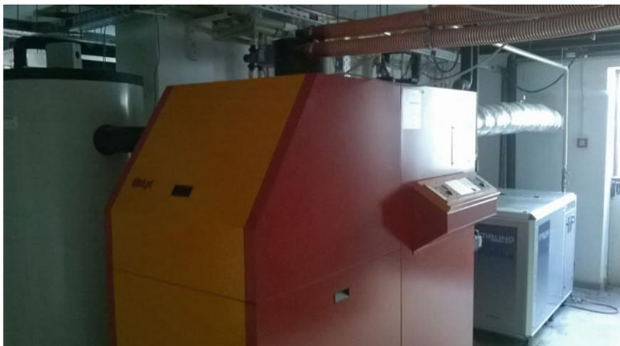
**Picture 3** Pellet boiler and Stirling engine
