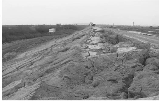
Figure 2. Photo (1) from site of instability embankment.
