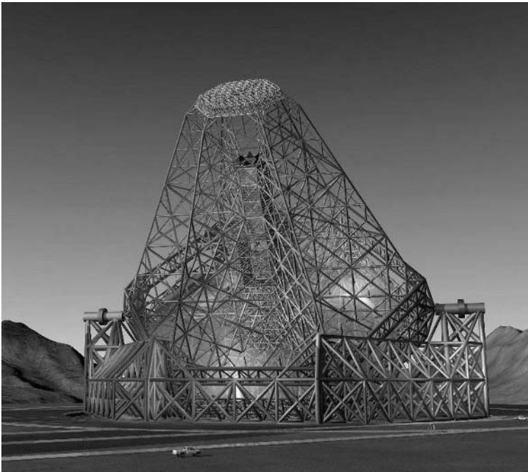
Fig. 11.1. OWL (the Overwhelmingly Large Telescope) is a European design for a 100m telescope. It uses large-scale replication of similar optical and mechanical components (Gilmozzi 2004, Dierickx et al. 2004). ( Courtesy European Southern Observatory. )
