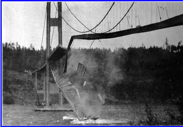
FIGURE 3.88 Collapse of Tacoma Narrows Bridge (November 7, 1940) due to wind loads. (From Smith, D., A case study and analysis of the Tacoma Narrows Bridge failure, 99.497 Engineering Project, Department of Mechanical Engineering, Carleton University, Ottawa, Ontario, Canada, March 29, 1974.)
