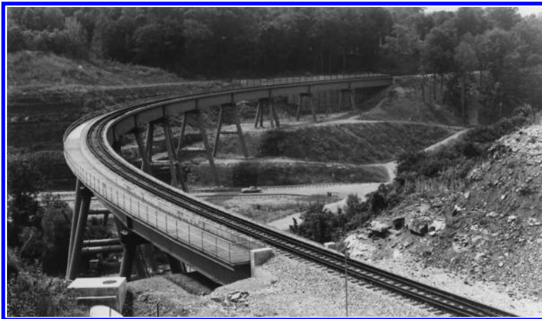
FIGURE 6.4 A curved steel plate girder railroad bridge (The Gulf Bridge, Lock, New York). (Courtesy of AISC, Chicago, IL.)
