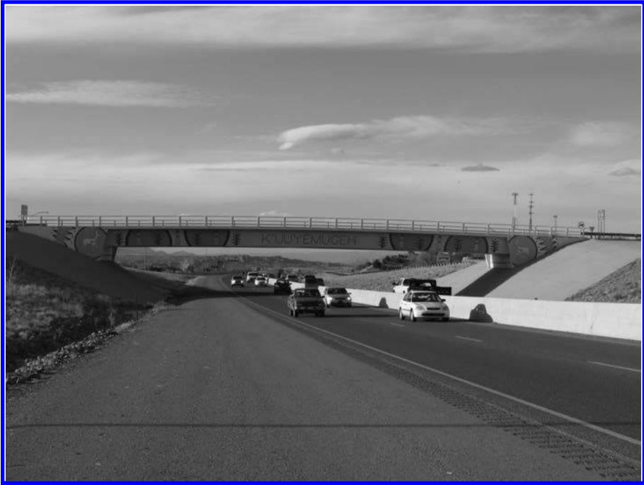
FIGURE 2.1 A typical single-span highway bridge. (Photo by author.)
