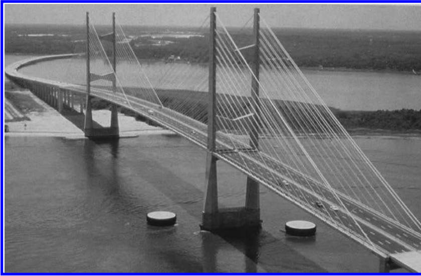
FIGURE 3.84 Dolphins protection system for the Dam Point cable-stayed bridge near Jacksonville, Florida. (Courtesy of Florida Department of Transportation, Jacksonville, FL.)
