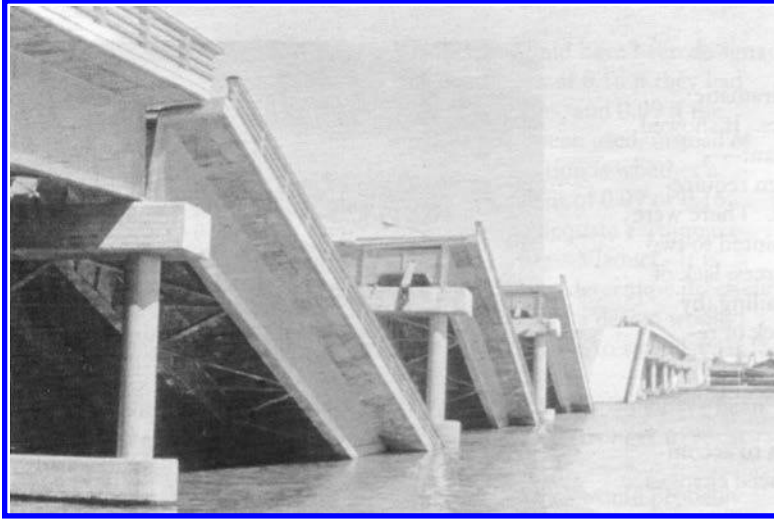
FIGURE 3.98 Collapse of the Showa Bridge during the 1964 Niigata, Japan, earthquake. Two piers in the middle of the river failed, causing three spans to drop (front of the photo). Two other spans slipped off piers that remained upright (back of the photo).
