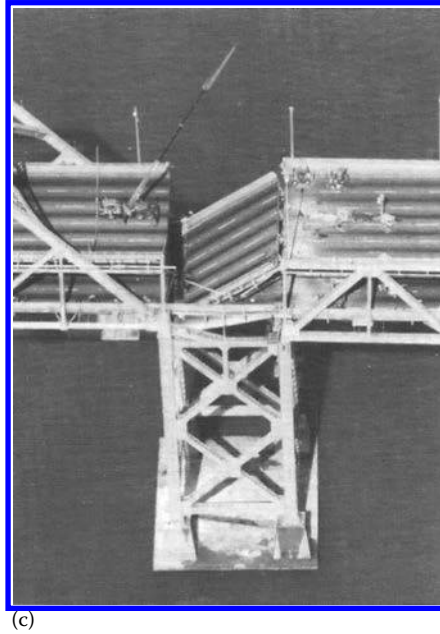
FIGURE 3.99 (Continued) Collapse of the upper and lower decks of the East Bay Bridge, San Francisco, during the October 17, 1989, M 7.1 Loma Prieta earthquake: (c) aerial view of the collapsed upper and lower decks.
