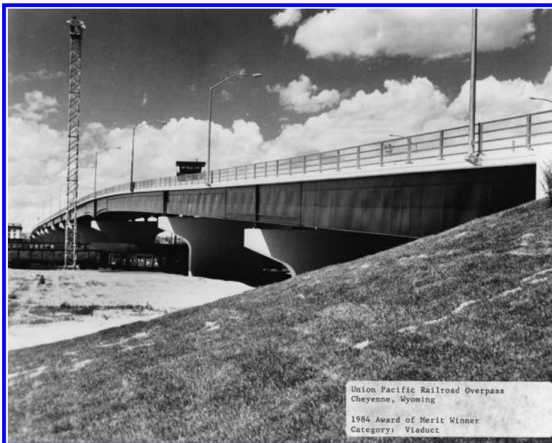
FIGURE 6.41 Union Pacific Railroad Overpass, Cheyenne, Wyoming. Longitudinal stiffeners are oriented horizontally, parallel to the compression flange (top flanges between the span and bottom flanges over the support). The longitudinal stiffeners are oriented parallel to the haunched curved bottom flange (in compression) over one of the supports on the left side of the bridge. (Courtesy of American Institute of Steel Construction, Chicago, IL.)
