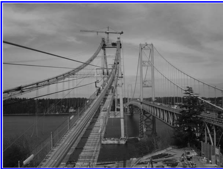
FIGURE 2.7 A suspension bridge (right: Tacoma Narrows Bridge 2 completed in 1950, left: Tacoma Narrows Bridge 3, under construction in 2007). (Photo by author.)
