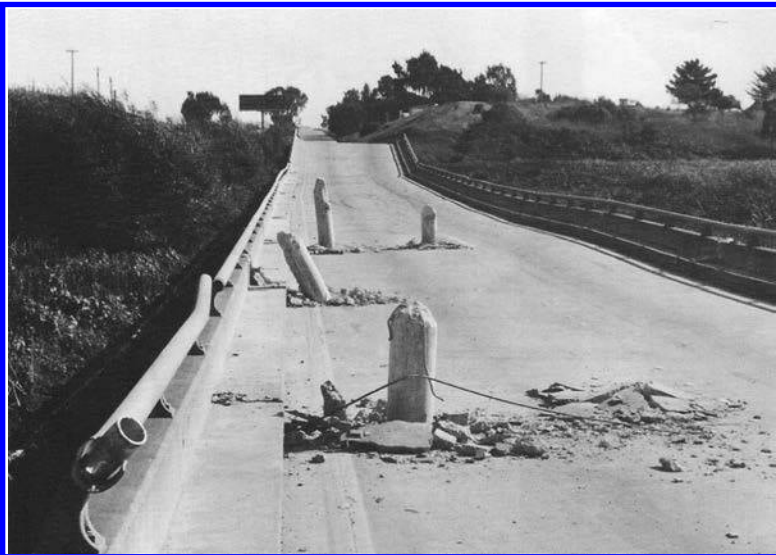
FIGURE 3.92 Collapse of the Struve Slough Bridge, Watsonville (California), with concrete support columns punching through the bridge deck like toothpicks, during the October 17, 1989, M 7.1 Loma Prieta (California) earthquake.
