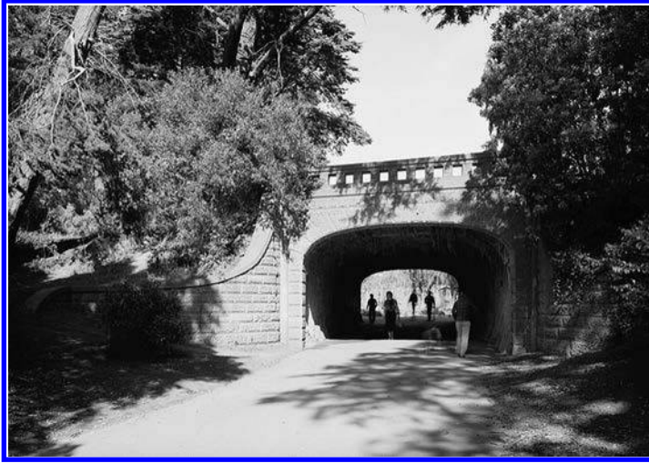
FIGURE 5.1 Lake Alvard Bridge, San Francisco Park, California, the oldest concrete bridge built in the United States in 1889 by Ernest L. Ransome, an innovator in reinforced concrete design, mixing equipment, and construction systems. The bridge, which arches over a pedestrian entrance to San Francisco's Golden Gate Park, was constructed as a single arch 64 ft (20 m) wide with a 20 ft (6.1 m) span. Ransome is believed to have used his patented cold-twisted square steel bar for reinforcement, placed longitudinally in the arch and curved in the same arc. The face of the bridge was scored and hammered to resemble sandstone; the interior features concrete stalactites (some of which have subsequently grown due to redeposition of limestone from the concrete). This bridge was designated a civil engineering landmark by the American Society of Civil Engineers in the 1970s. (From Library of Congress—Alvard Lake Bridge: General View Looking East.)
