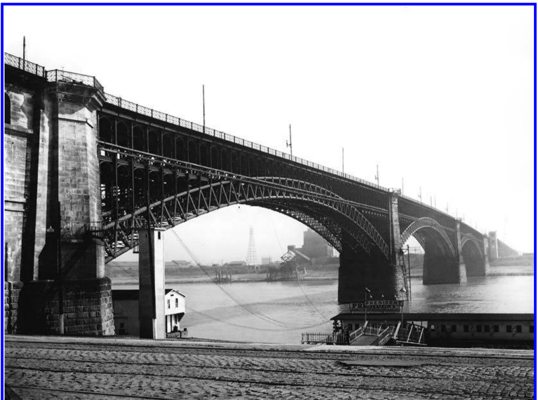
FIGURE 2.4 The Eads Bridge, St. Louis, MO. Built by James Eads (1820–1887) and opened to traffic on July 4, 1878, the construction of this bridge was a milestone in the history of bridge engineering. This triple-arch bridge (502-520-502 ft) carries two railroad tracks on its lower deck and highway traffic on the upper deck. The three arches are fixed ended, and thus indeterminate. When built, these arches were the first ever to span distances of over 500 ft. The arches marked the first ever use of steel in bridge building, as well as the first ever use of tubular steel members for chords. See Taly (1998) for more on this great bridge. (Courtesy of AISC, Chicago, IL.)
