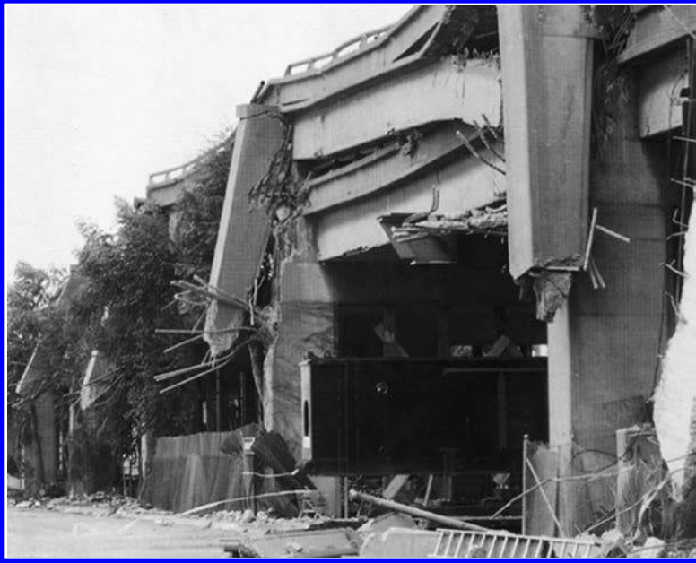
FIGURE 3.91 Spectacular collapse of the double-deck Cypress Viaduct during the Magnitude 7.1 1989 Loma Prieta, California, earthquake. A large portion of this viaduct collapsed during the earthquake killing 41 people. (From The Governor's Board of Inquiry on the 1989 Loma Prieta Earthquake, Competing against Time: Report to Governor George Deukmejian from the Governor's Board of Inquiry on the 1989 Loma Prieta Earthquake , State of California, Office of Planning and Research, San Francisco, CA, 1990.)
