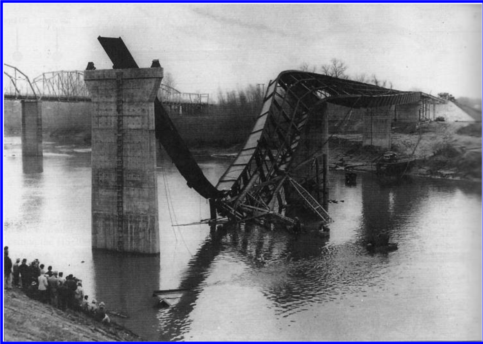
FIGURE 6.14 Collapse of the Brazos River Bridge, Brazos, Texas, during erection of the 973 ft, continuous steel plate girders that support the roadway. The failure was initiated by overstress of the connections between the web and flange during erection. (Courtesy of Simpson, Gumpertz, and Heger, Inc.)
