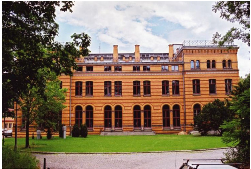
Fig. 13 Central Building, Prussian Geodetic Institute, Potsdam Telegraphenberg, Geoforschungszentrum Potsdam
