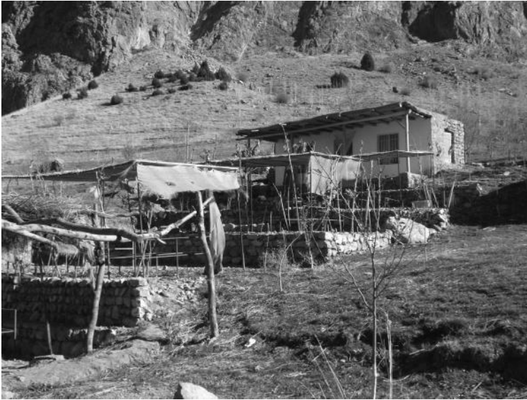
FIGURE 20.11 An existing old restaurant.
