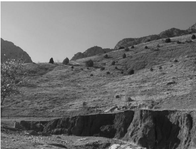
FIGURE 20.14 Destroyed river banks.
