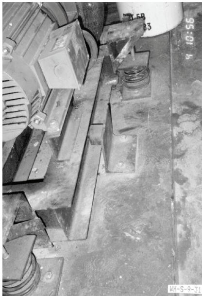
Figure 6.6: Bumpers should be included to limit the movement of vibration isolated equipment. Uplift restraints should also be provided.
