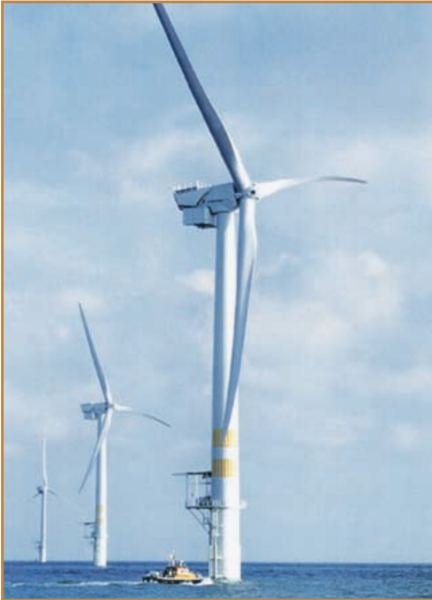
This is the Arklow Bank, Ireland Offshore Wind Farm, located about 6 miles (10 km) off the coast of Arklow, Ireland. This wind park is the world's first commercial application of offshore wind turbines that is more than 3 megawatts in size, and Ireland's first offshore wind facility. (Photo courtesy of National Oceanic and Atmospheric Administration)
