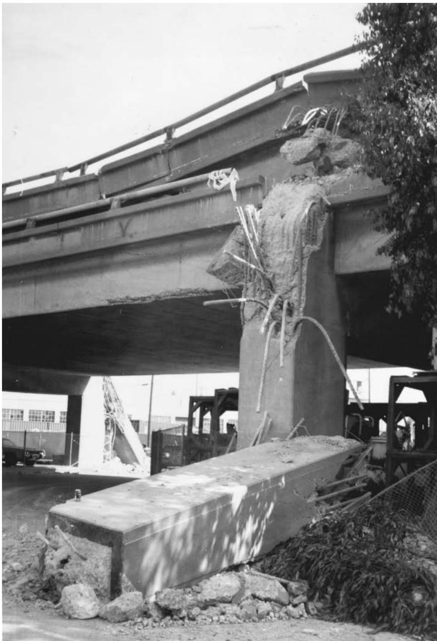
**Figure 68** *Collapsed bridge on Interstate 880 in San Francisco from the October 17, 1989 Loma Prieta earthquake, Alameda County, California.*
