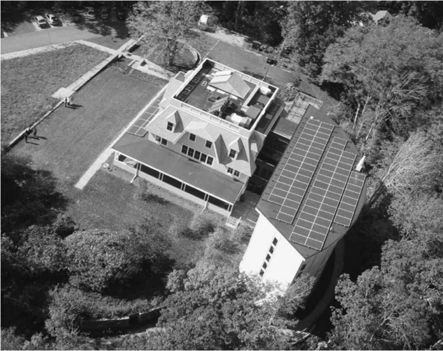
Figure 4.3 A group of architects took an interest in the building and one of them used a kite-borne camera to take this photograph showing the arrays of photoelectric panels, one on the roof of the porch of the original building and the other on the roof of the new wing. Three hot water panels are visible on the roof of the main building. (Photo courtesy of Charles C. Benton, U. California, Berkeley)
