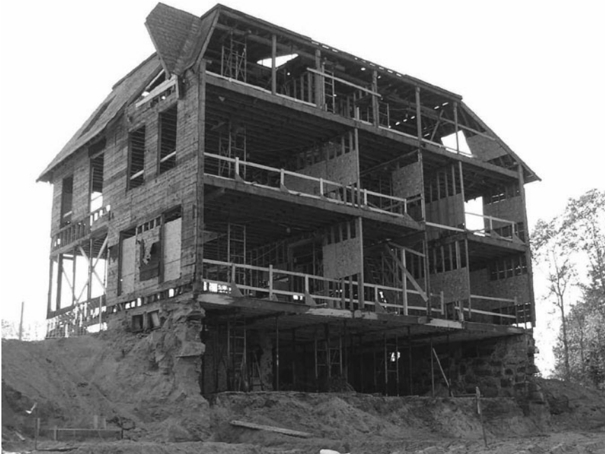
Figure 3.3 Deconstruction of Hilltop House. The structure required a little more renovation than anyone had anticipated.
