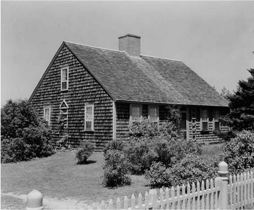
Figure 3.2 A Cape Cod cottage. The central chimney supported a fireplace in each room and the chimney's mass, once heated, lent stability to the heating system for the whole house. (Jonathan Kendrick House, State Highway, South Orleans. Historic American Buildings Survey, Arthur C. Haskell, Photographer, 1935. HABS, Mass 1-ORLS.1. Library of Congress)
