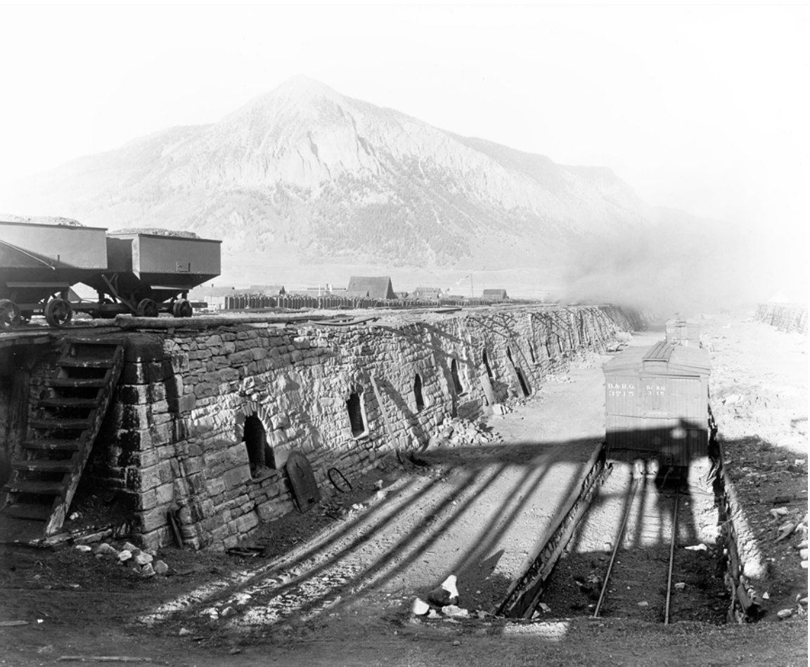
Figure 14. Coke Ovens at Crested Butte. Essentially a company town of the Denver & Rio Grande Railway, Crested Butte and its ovens extended Pueblo's manufacturing interests to western Colorado. Boxcars carry coking coal. The smoke from the ovens almost obscures the 12,172-foot butte in the background. Photograph by George L. Beam. Courtesy of Denver Public Library, Western History Collection.
