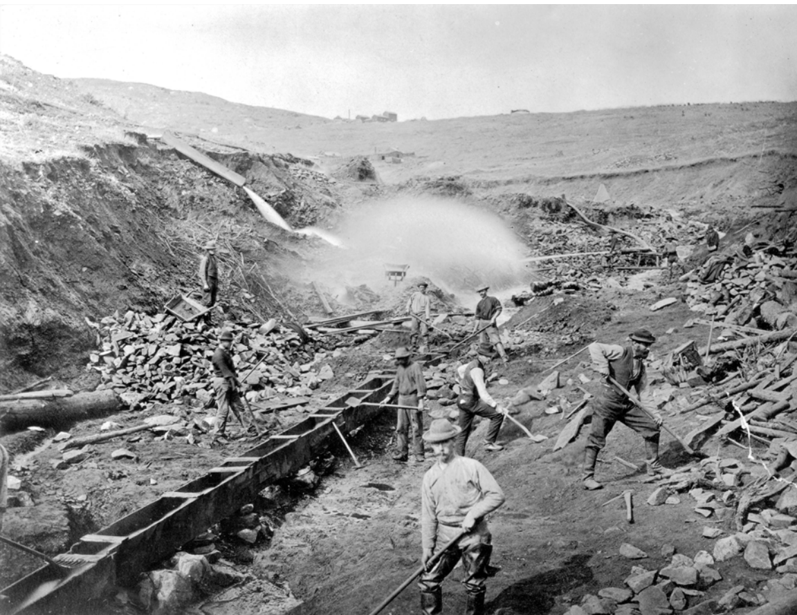
Figure 1. Early Placer Mining. Placer miners operating sluices near Black Hawk, Colorado, illustrate the use of water and wood resources in what became increasingly more complex hydraulic operations. Courtesy of Denver Public Library, Western History Collection.
