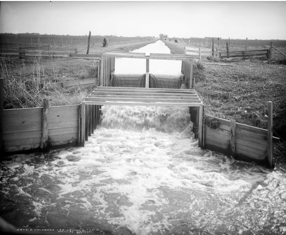
Figure 6. Plains Irrigation Ditch. Viewed from downstream, water flows through the wood-slatted sluice in this irrigation ditch typical of Colorado's eastern plains. Fenced farmland occupies the flat, nearly treeless horizon. Photograph by Louis Charles McClure. Courtesy of Denver Public Library, Western History Collection.
