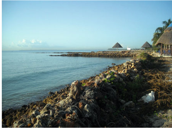
Fig. 3.11 Improvised groins at Mbezi Beach area Dar es Salaam (photograph taken by Dionis Rugai in June 2011)
