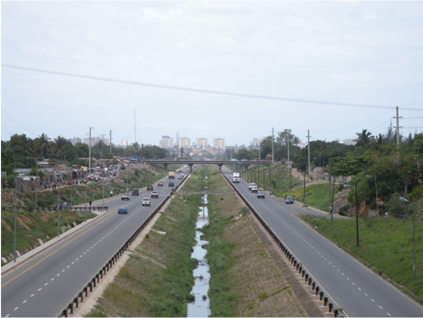
Fig. 13.2 Maputo, 5 Nov. 2011. A primary rainwater drainage canal along Kahunda Street, properly maintained (Tiepolo 2011)
