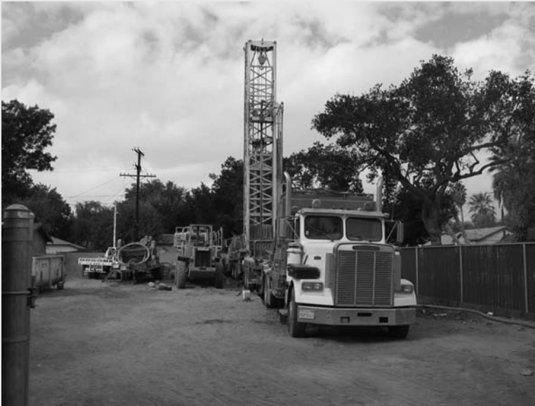
Air rotary drilling rig
