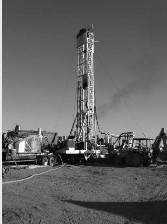
Mud rotary drilling rig
