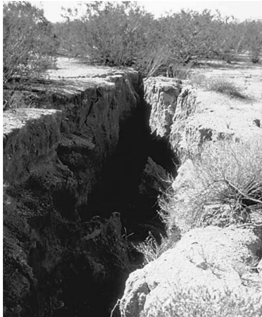
FIGURE 6.5 Fissure has been attributed to land subsidence related to groundwater pumping in the Antelope Valley area, California. (Source: U.S. Geological Survey)
