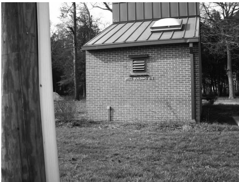
FIGURE 1.1 Well house, Bethany Beach, Delaware.
