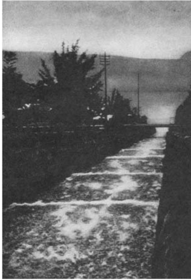
Figure 6.15 Roll waves, looking downstream (The Grünbach, Switzerland). From Stoker (1957).
