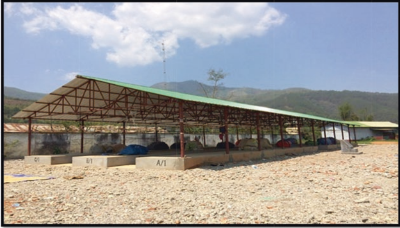
Fig. 5 Interim market space for women vendors built after the earthquake in Saikul
