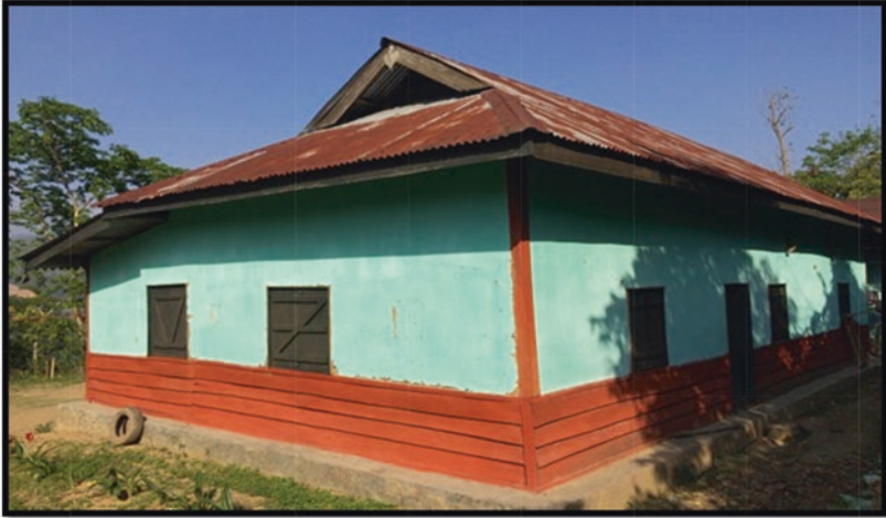
Fig. 4 A traditional house (wooden frame, with bamboo mat infill walls and CGI sheet roofing) with no noticeable damage in Noney, one of the nearest locality from earthquake epicentre
