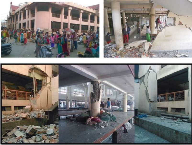
Fig. 2 Ima Market in Imphal in April 2016 and partial damage of the same due to the M6.7 earthquake of 4 January 2016 ( Source Chandan Ghosh and www.nelive.in )
