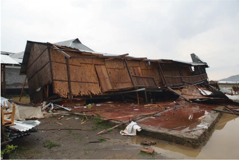
Fig. 3 One of the many houses in Khominthang area of Lamka town damaged by hailstorm in May 2013
