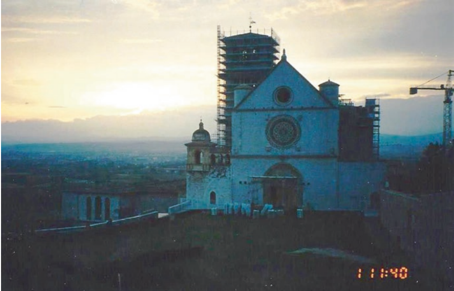
Fig. 7.1 SaF: rebuilding a building
