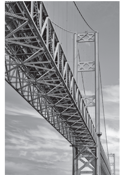
Photo 4.1: Reconstructed Tacoma Narrows bridge showing trusses used to stiffen the roadway floor system. See original bridge in Photo 2.2.
