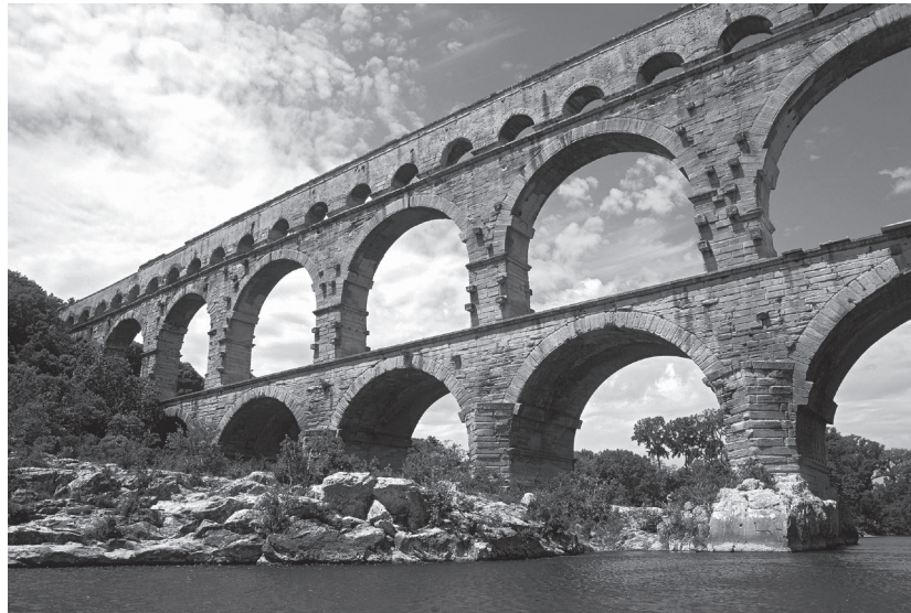
Photo 1.2: Romans pioneered in the use of arches for bridges, buildings, and aqueducts. Pont-du-Gard. Roman aqueduct built in 19 B.C. to carry water across the Gardon Valley to Nîmes. Spans of the first- and second-level arches are 53 to 80 ft. (Near Remoulins, France.)
