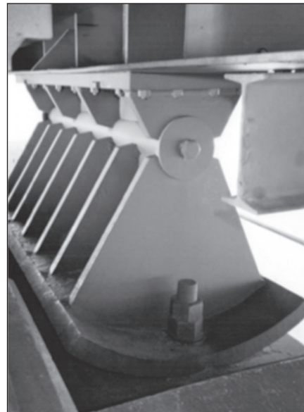
Photo 3.2: Roller support for the San Diego-Coronado Bridge.
