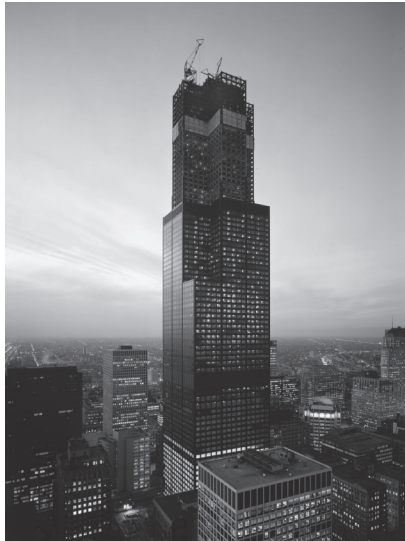
Photo 5.2: Fazlur Rahman Khan developed the innovative bundled tube structure concept for the Willis Tower, commonly known as Sears Tower, in Chicago. The building is composed of 9 (3 by 3) tubes rising up to different heights. This concept continues to influence the construction of modern super-tall buildings.
