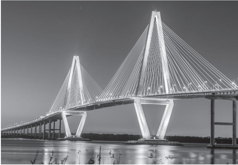
Photo 6.2: Cable-stayed bridge over the Cooper River in Chareleston, South Carolina. © iStock/Getty Images Plus
