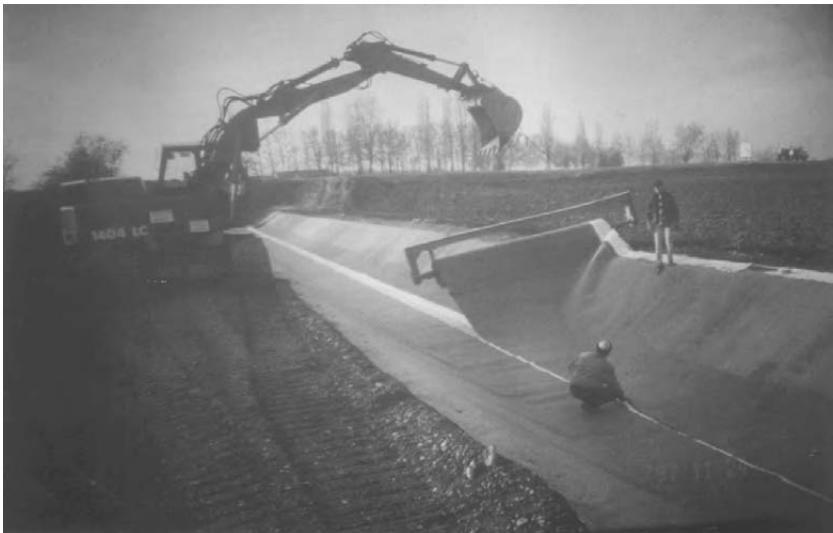
Figure 9.19 The Mulhouse (France) canal: geomembrane-geotextile composite installation (after Duquennoi, 2002).
