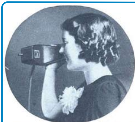
"Television monocle" in use. It works like a hand phone set
