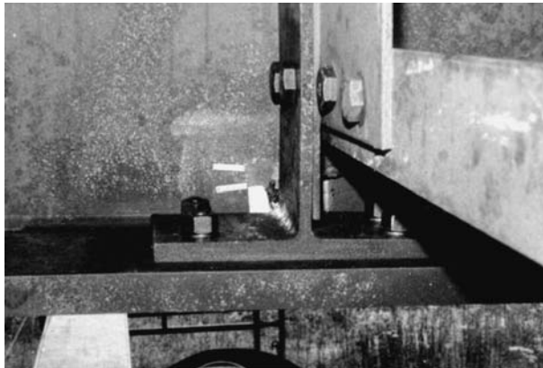
Figure 14 Retrofitting by connection stiffening.
