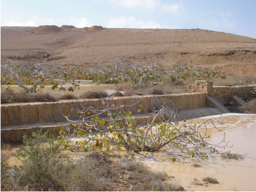
Fig. 6.21 Water infrastructure in the wadi bed for agriculture development (figs in this case)
