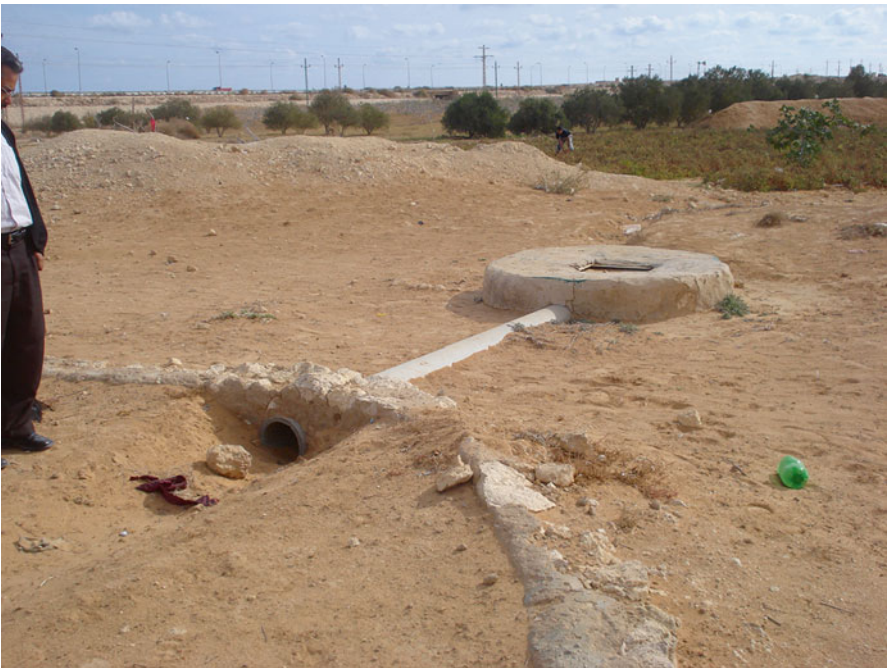
Fig. 6.20 Cistern built by the Matruh Resource Management Project for a Bedouin family near Nagamish wadi
