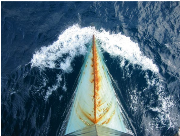
Fig. 1.7 Corrosion on the bow of an oil tanker (Photo by Haus)
