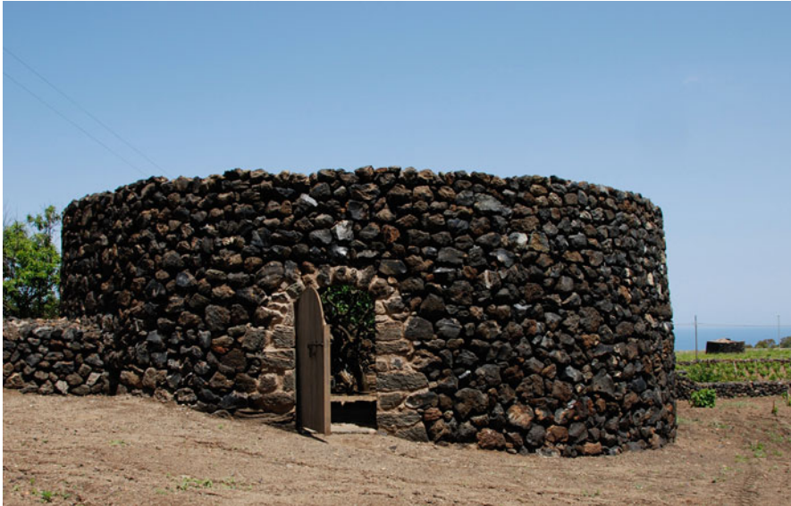
Fig. 1.14 The panteschi gardens on the island of Pantelleria (for this study area, see the Sicily chapter), are an important instance of FAO's Globally Important Agriculture Heritage Systems (GIAHS), partly because they are an example of adaptation to a hot climate. Inside each of these circular dry-stone buildings a single citrus tree is planted, which grows without needing any irrigation thanks to the microclimate created inside the garden. If planted outside, the tree would soon succumb to the windy and dry climate of the island
