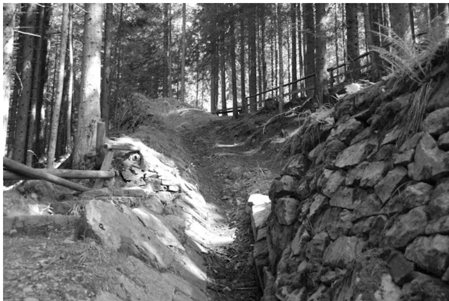
Fig. 10.1 Part of a stone cava in Val Cadino. These traditional transportation systems are a unique feature of this Alpine area
