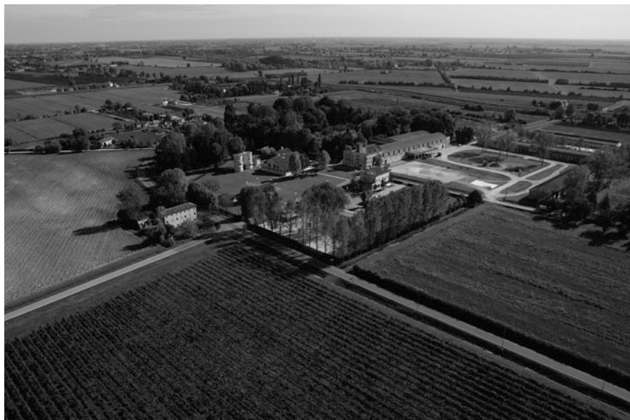
Fig. 12.7 The central buildings of the Ca' Tron farm are the elements showing the highest degree of persistence and integrity
