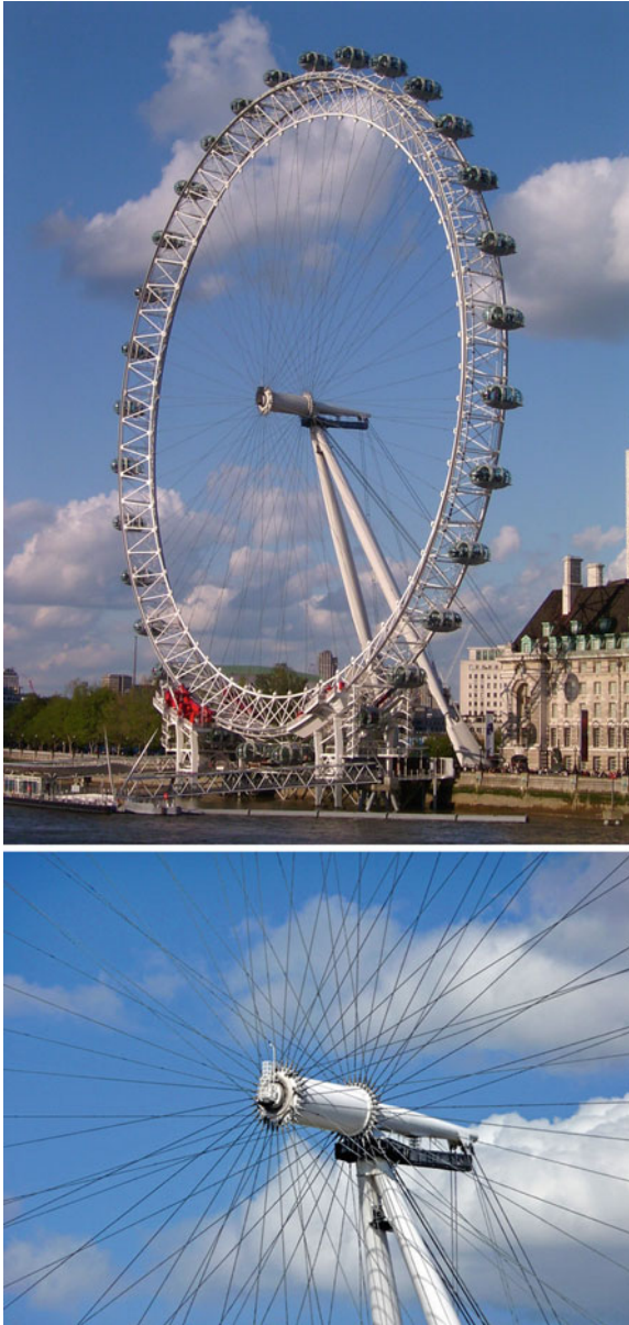
Fig. 1.20 The London Eye observation wheel ( upper ) with the rim supported by tensioned steel cables ( lower , photo by Christine Matthews). The wheel works like a huge spoked bicycle wheel
