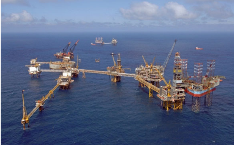
Fig. 16.4 Several offshore jackets and tripod structures connected by bridges at Ekofisk fields of North Sea (courtesy of Aker Solutions)
