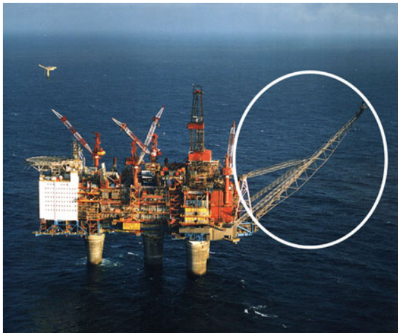
Fig. 16.9 A flare boom (marked with a circle) installed on a gravity based offshore structure in the North Sea (courtesy of Aker Solutions)
