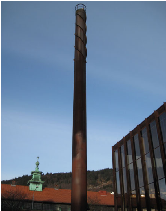
Fig. 1.18 A spiral strake installed on the upper part of a chimney to diminish VIV (photo by Jing Dong)
