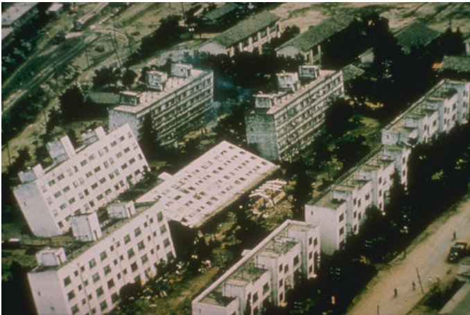
Fig. 1.4 Appearance of soil liquefaction after the 7.4 magnitude Niigata earthquake, Japan June 16, 1964 (courtesy of National Geophysical Data Center)
