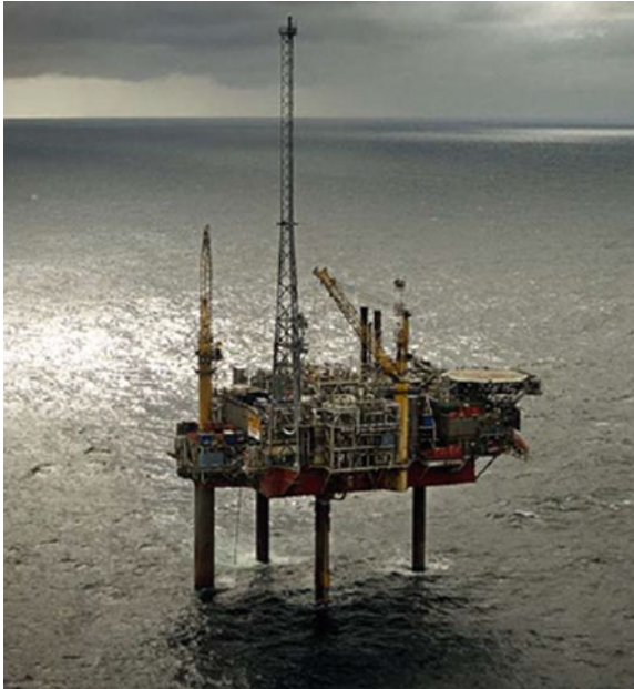
Fig. 13.12 The Siri jack-up structure located in the North Sea (courtesy of Dong Energy Denmark)
